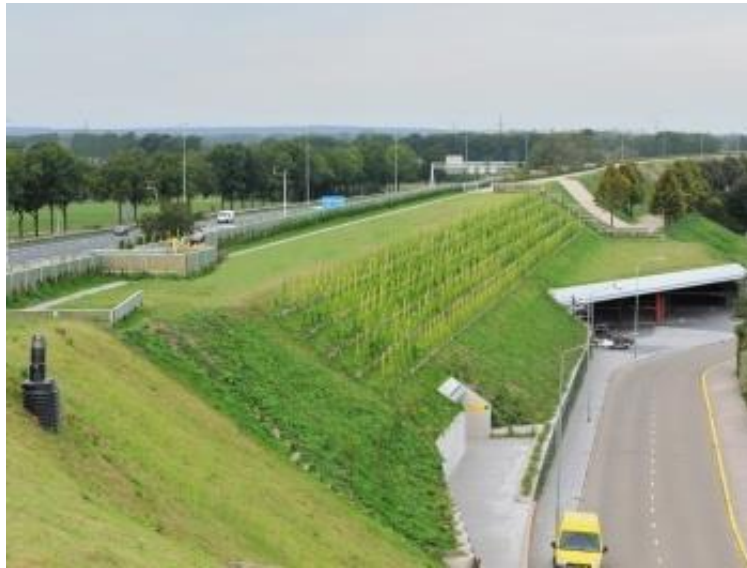
Figure 3: the parking garage of the CineMec in Ede is built into the noise barrier for the A12 motorway in the Netherlands.
