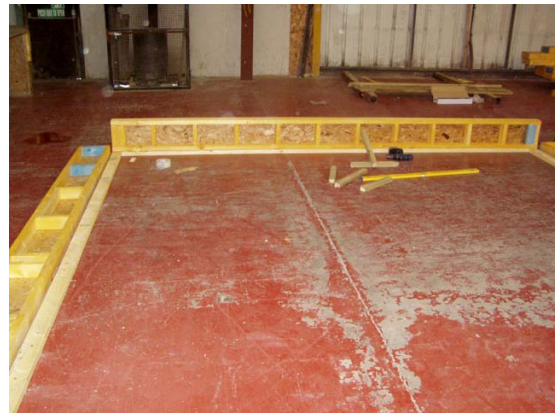
(b) Wall panels fixed onto the solid frame
