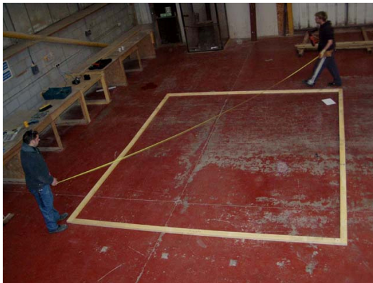
(a) Wall plates assembled to frame
