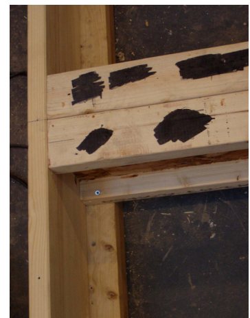
(b) Detail of double joist at the supports
