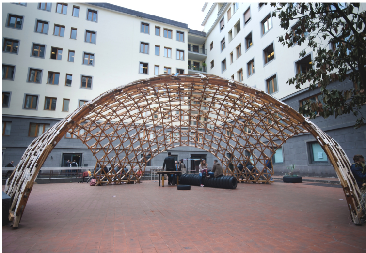
Figure 10: Toledo timber gridshell 2.0. Completed structure (Photos courtesy - Daniele Lancia).
