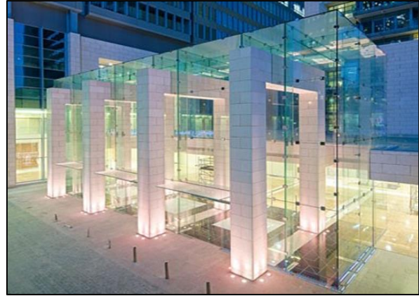
Figure 1-2: Entrance to Daman Building, Dubai - ( www.malishevengineers.com ).
