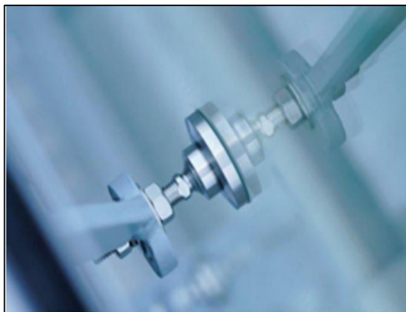
Figure 2-7: Glass point-fixing with modern adhesive [13].
