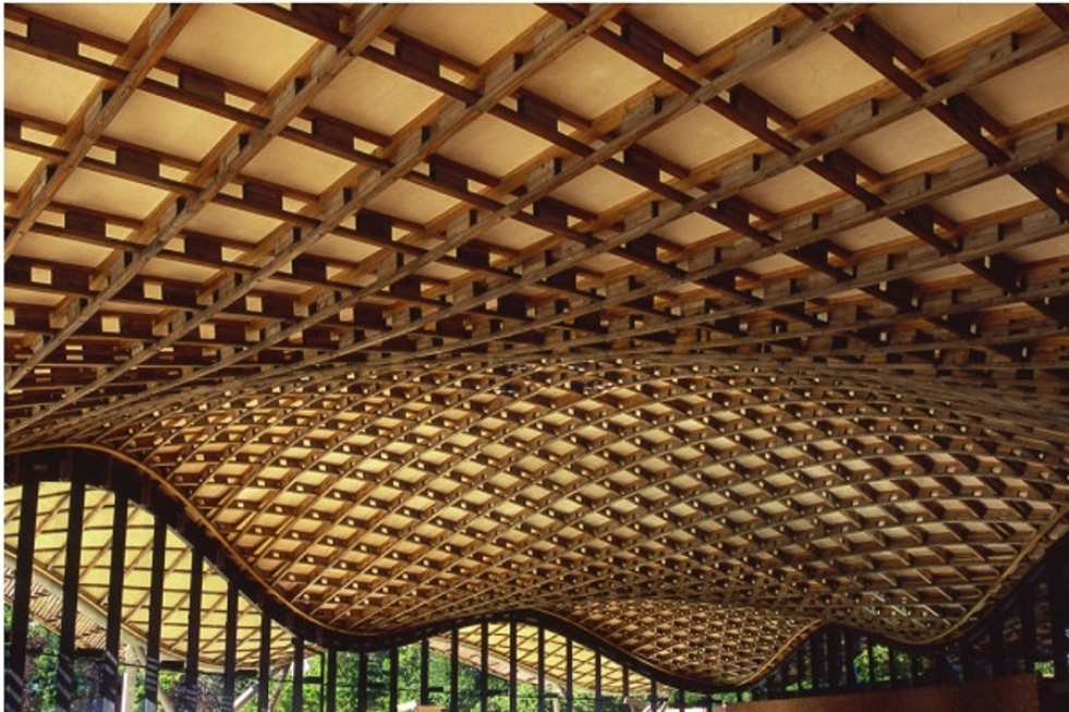
Figure 1.11: Savill Garden grid-shell, Surrey, UK, 2006: (a) External view; (b) Internal view. Images source: http://glennhowells.co.uk (Accessed: 23/04/2015).
