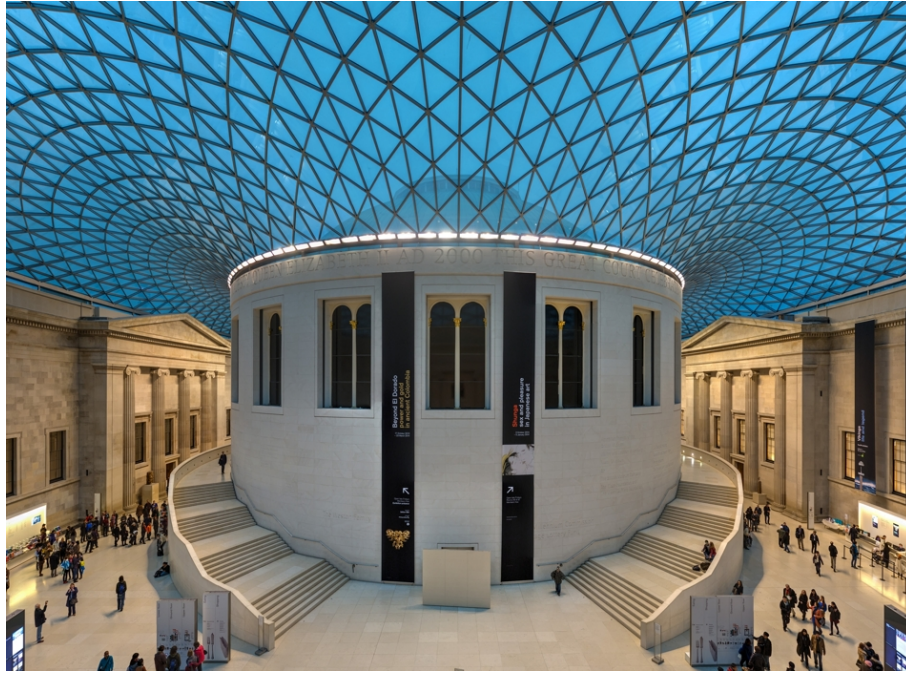
Figure 1.1: Great court grid-shell roof at the British Museum. Photo by David Iloff. (License: CC-BY-SA 3.0).
