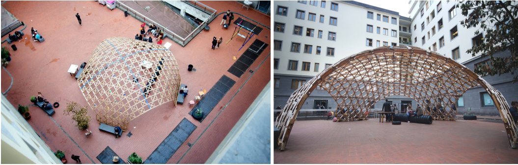
Figure 5.1: Toledo timber gridshell 2.0. Completed structure (Photos courtesy - Daniele Lancia).
