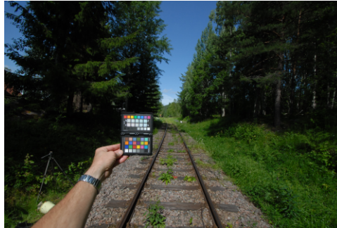
Figure 5.3: Overview Grycksbo: Railway section under investigation
