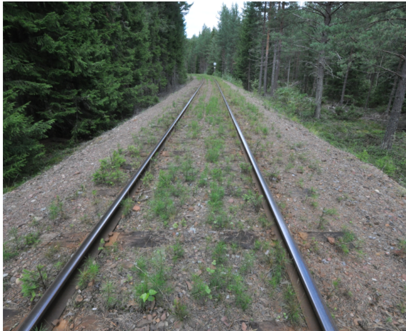
Figure 9.1: Overview, plot 200-204 (Oxberg, Sweden)
