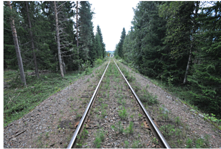
Figure 5.8: Overview of the sampled railway section (Oxberg, Sweden)
