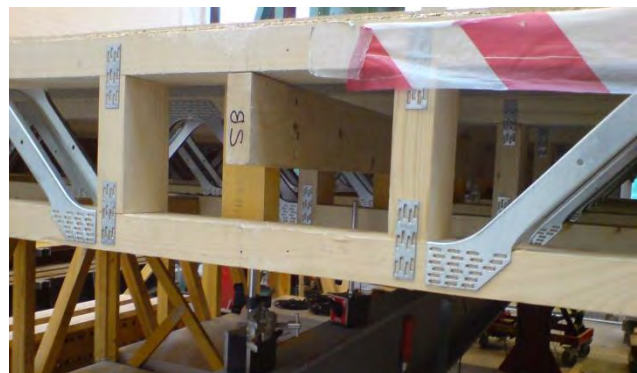
Figure 2: A TR26 strongback at mid-span in Floor E
