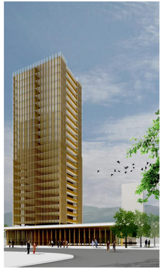
Glulam curtain wall and podium base
