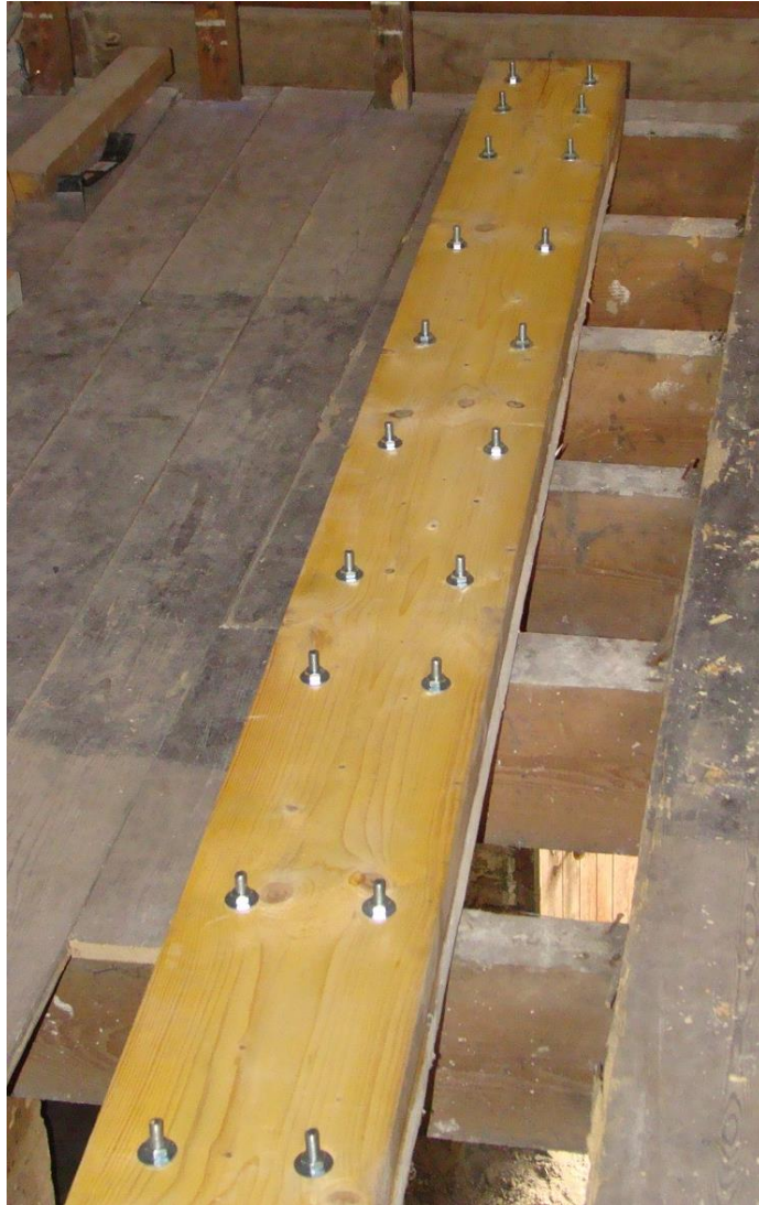
Bolted Flitch beam fabrication
