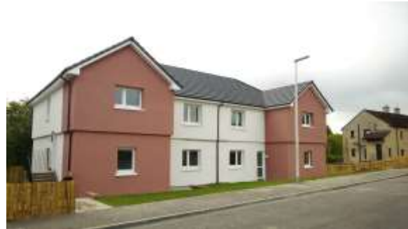
Figure 12. Lochore block As-built before occupation
