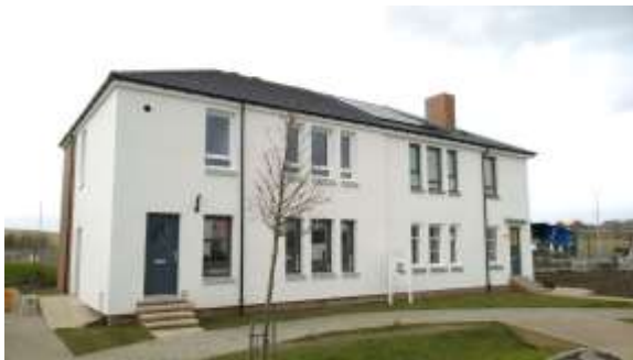
Figure 11. BRE block As-built for demonstration purposes.
