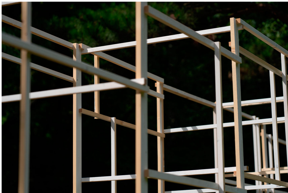
Figure 3. Photograph of 107\text{ m}^3 Pavilion, made of over 500 pieces of around 2 cm X 2 cm, both sides white painted lumber. Photograph courtesy of author.
