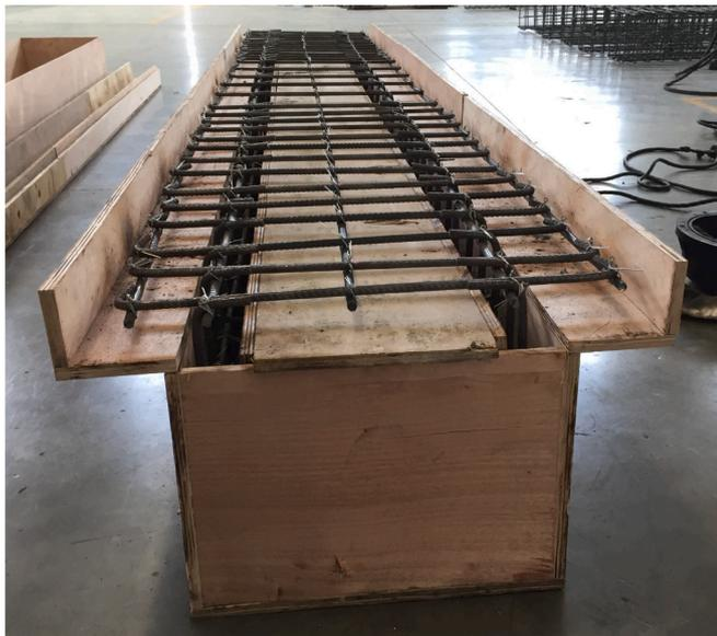
Fig. 4. Formwork for box girder concrete casting.
