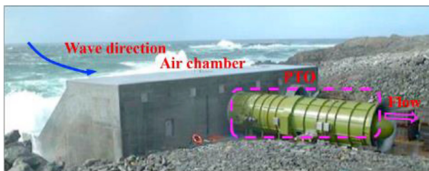
Fig. 9. Wavegen Limpet at Islay (Zhang et al. 2021).
