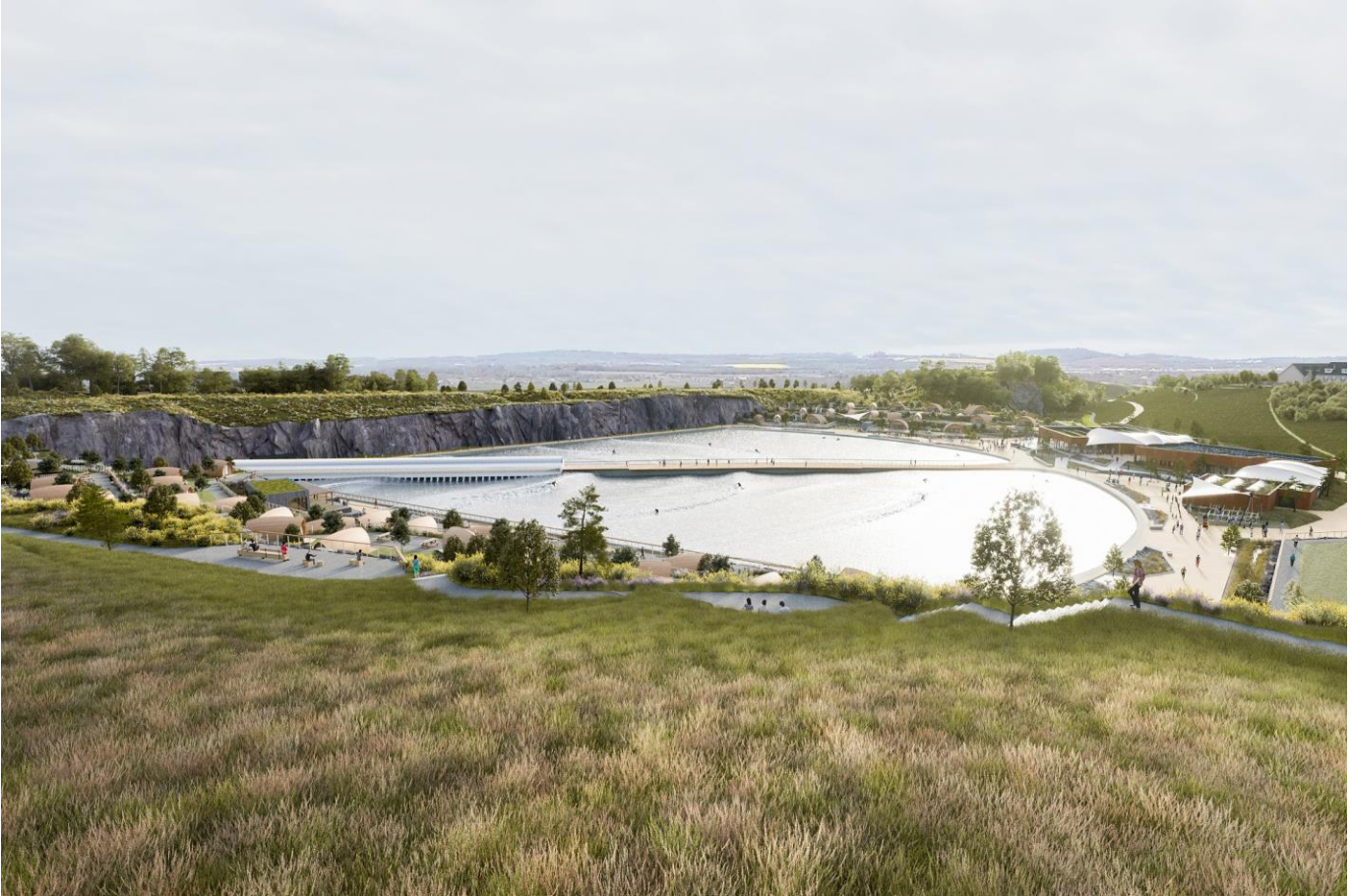
Computer generated rendering of proposed Wavegarden Scotland wave pool. Credit Tartan Leisure
