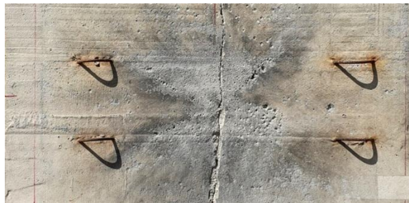
Figure 12a. Complete flexural failure pattern
