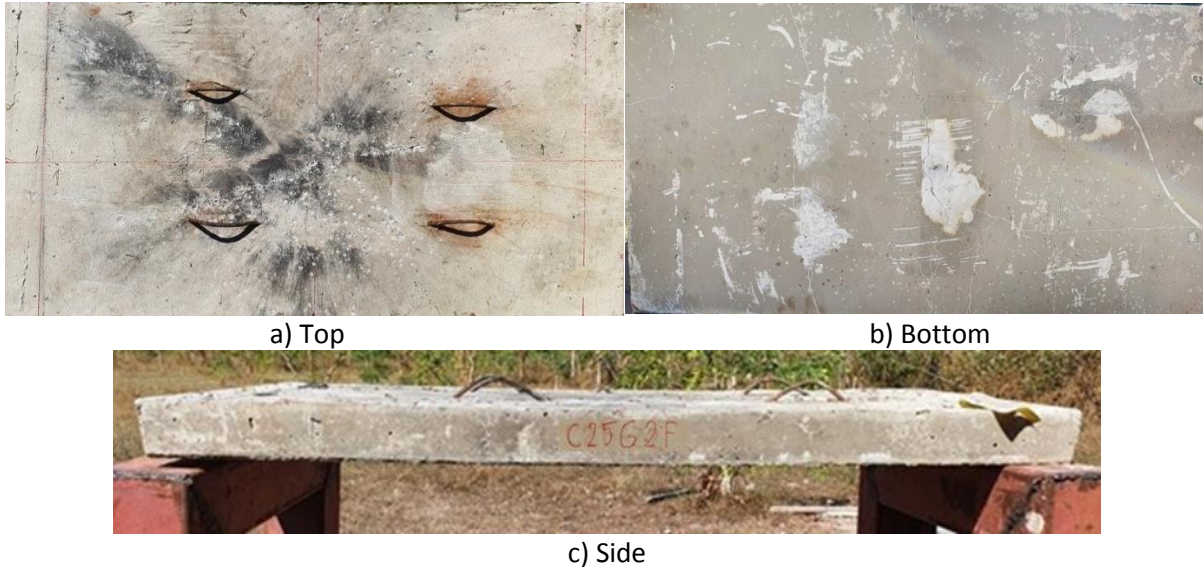
Figure 14. No major damage with microcracking pattern
