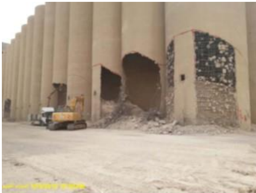
Figure 7 The Destruction of the Old Silos in Aqaba Port
