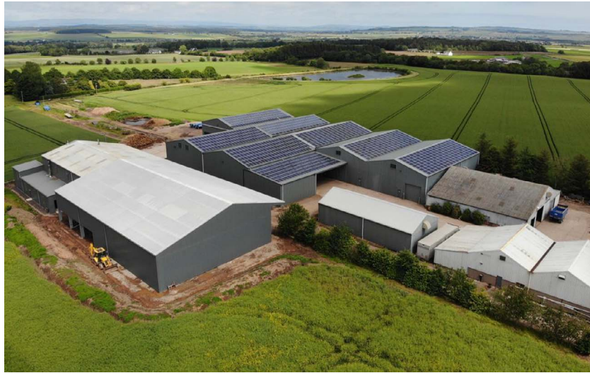
Figure 3. The 300kWp solar PV plant at Cononsyth, Arbroath, Scotland Note: The dull colored PV modules at the back of this picture were installed in year 2011. The brighter colored modules were installed in year 2019.
