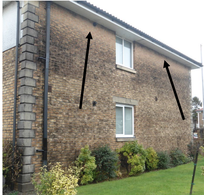
Figure 9: Heavy-Medium elevation demonstrating lack of growth beneath the eaves.
