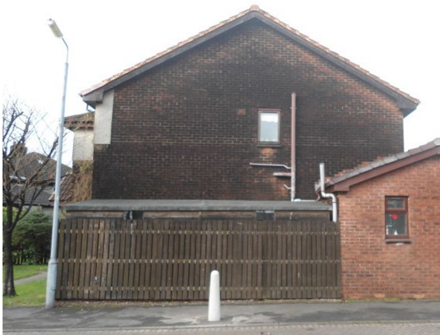
Figure 9: Heavy-Medium elevation demonstrating lack of growth beneath the eaves.
