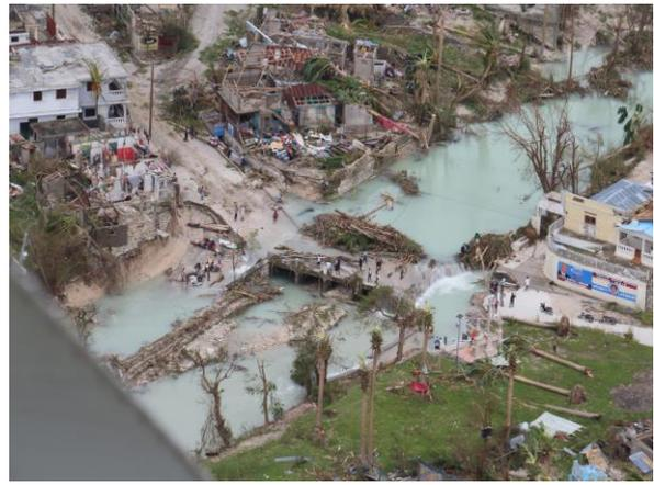
(d) Bridge collapsed by storm surge in Haiti (Source photo Tim Schandordff\_Mission Network.net)
