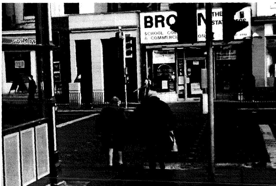
*Figure 1: View over a Puffin crossing. It can be seen that the Pelican's green man signal at the far side of the road is no longer present. This indication is instead given on the nearside (the uppermost of the two boxes mounted on the nearest signal pole).*
