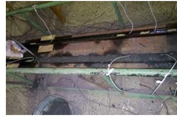
c) Pouring the concrete.
