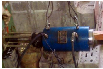
b) Prestressing the CFRP rods.
