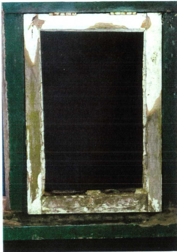
Fig. 2.3 (a) Fixed (top) end of window is less deteriorated as compared to open (bottom) end that is more exposed to flux of wind and moisture
