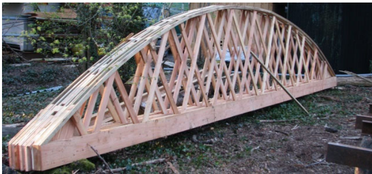
Figure C- 24 Sub-assembly system, Belfast truss [247]
