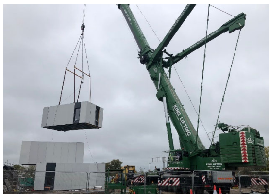
Figure 6-32 Dyson case study: On-site installation of units
