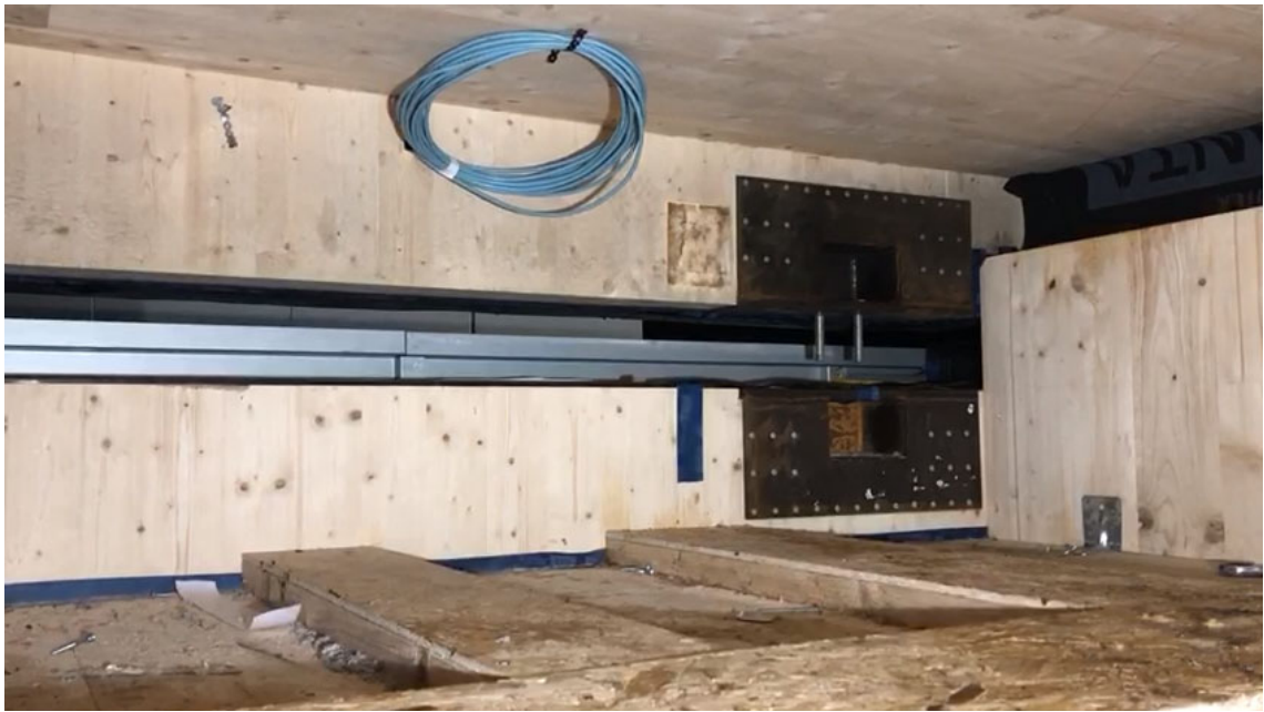
Figure 6-42 Dyson unit connection, internal view
