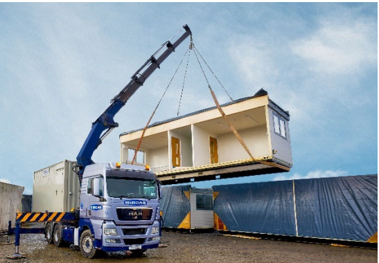
Figure C- 23 Volumetric modular system. From SiBCAS Ltd
