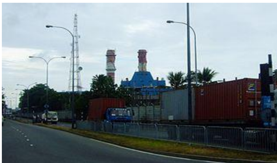
Fig 3-5 Kalanitissa Thermal power plant
