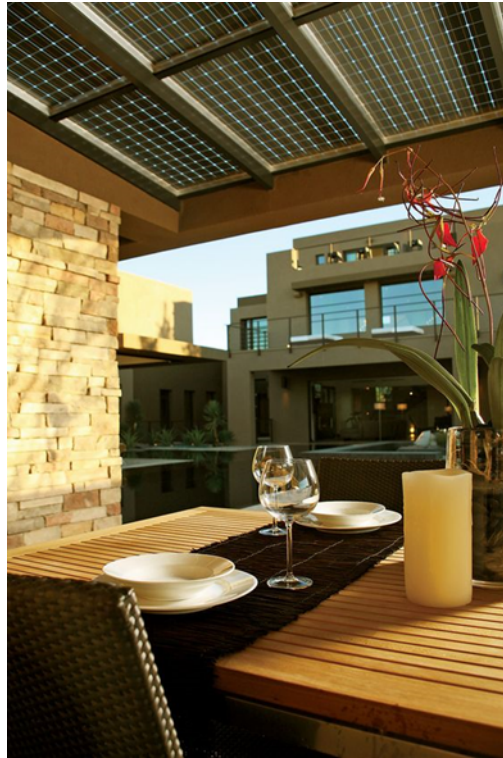
Figure 2. Skylight with monocrystalline PV modules [11].
