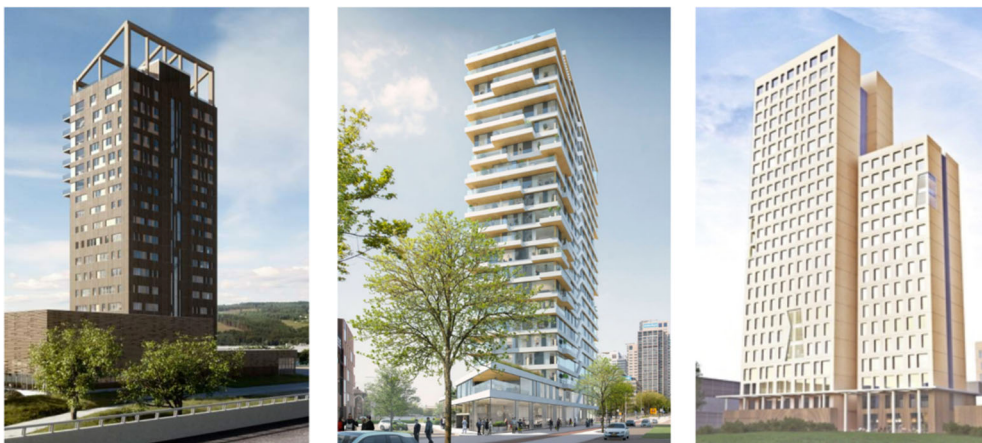
Figure 5. From left to right: Mjøsa Tower , Brumunddal; HAUT , Amsterdam; HoHo , Vienna, 2018 (Images from CTBUH, 2019)
