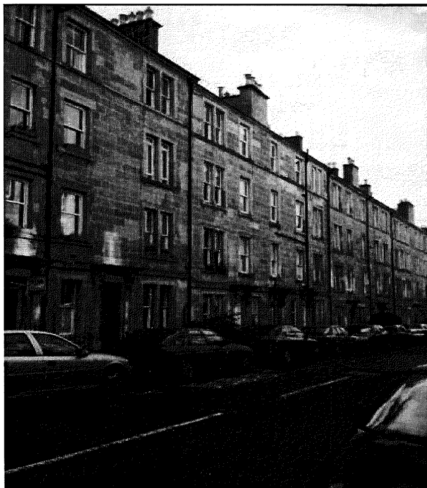
Figure 8.1. Bryson Road - an example of a tenement in the Dalry postcode sector
