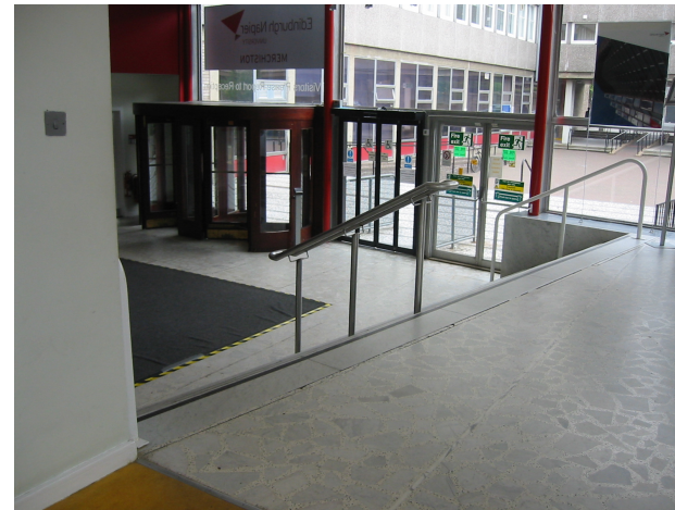
(d) Stairs at the end of the corridor towards the left.
