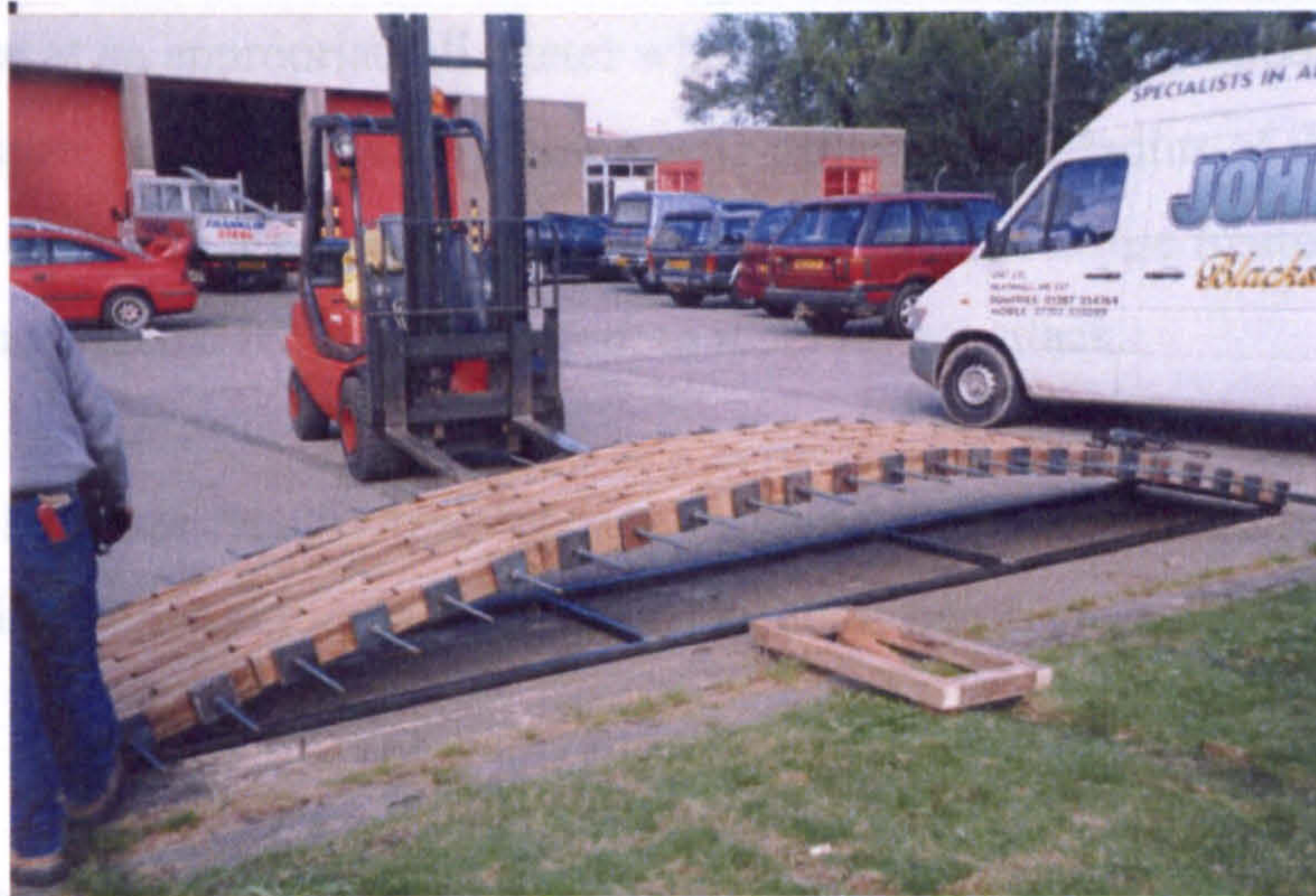
Fig 6.19 – First SLT arch
