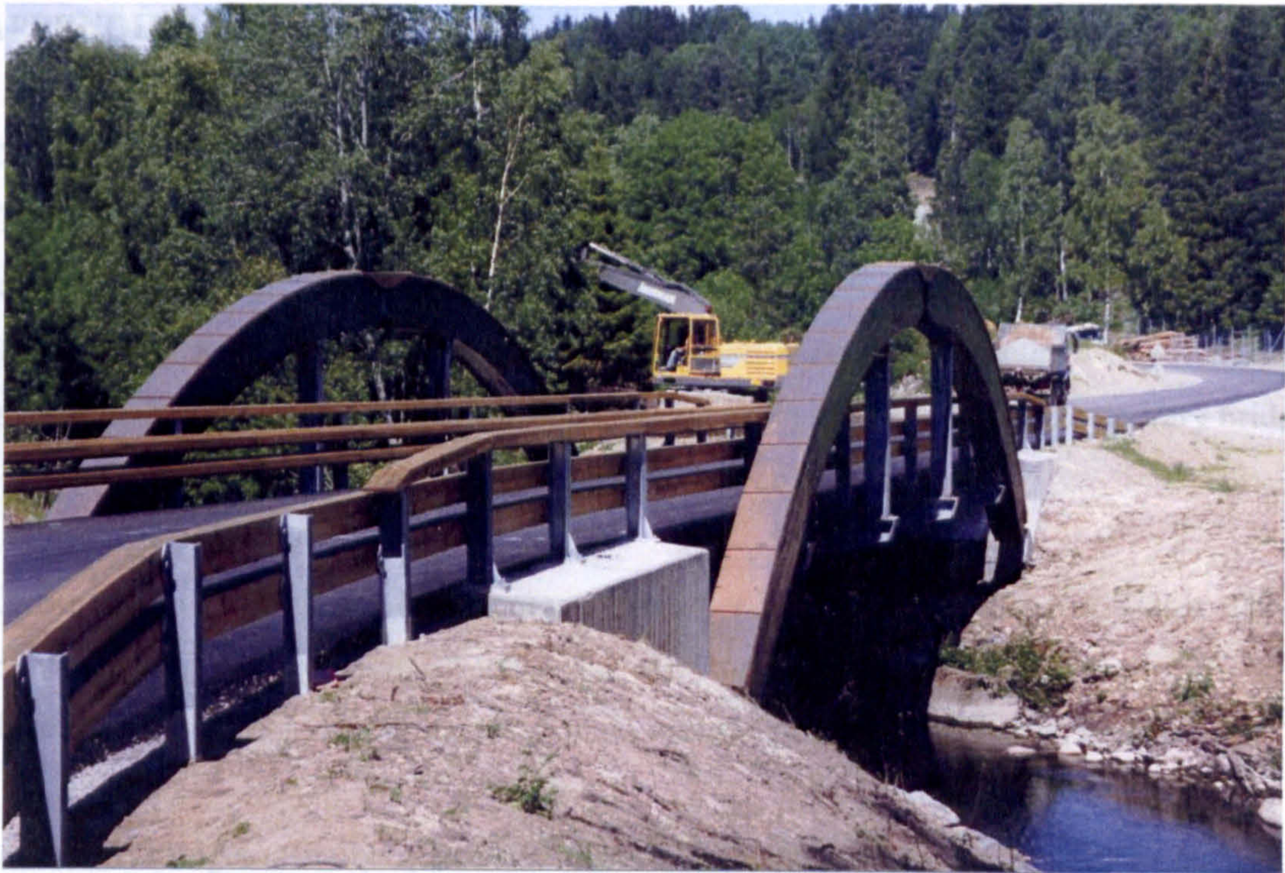
Norway – Glue laminated timber arch supporting SLT deck on trunk road
