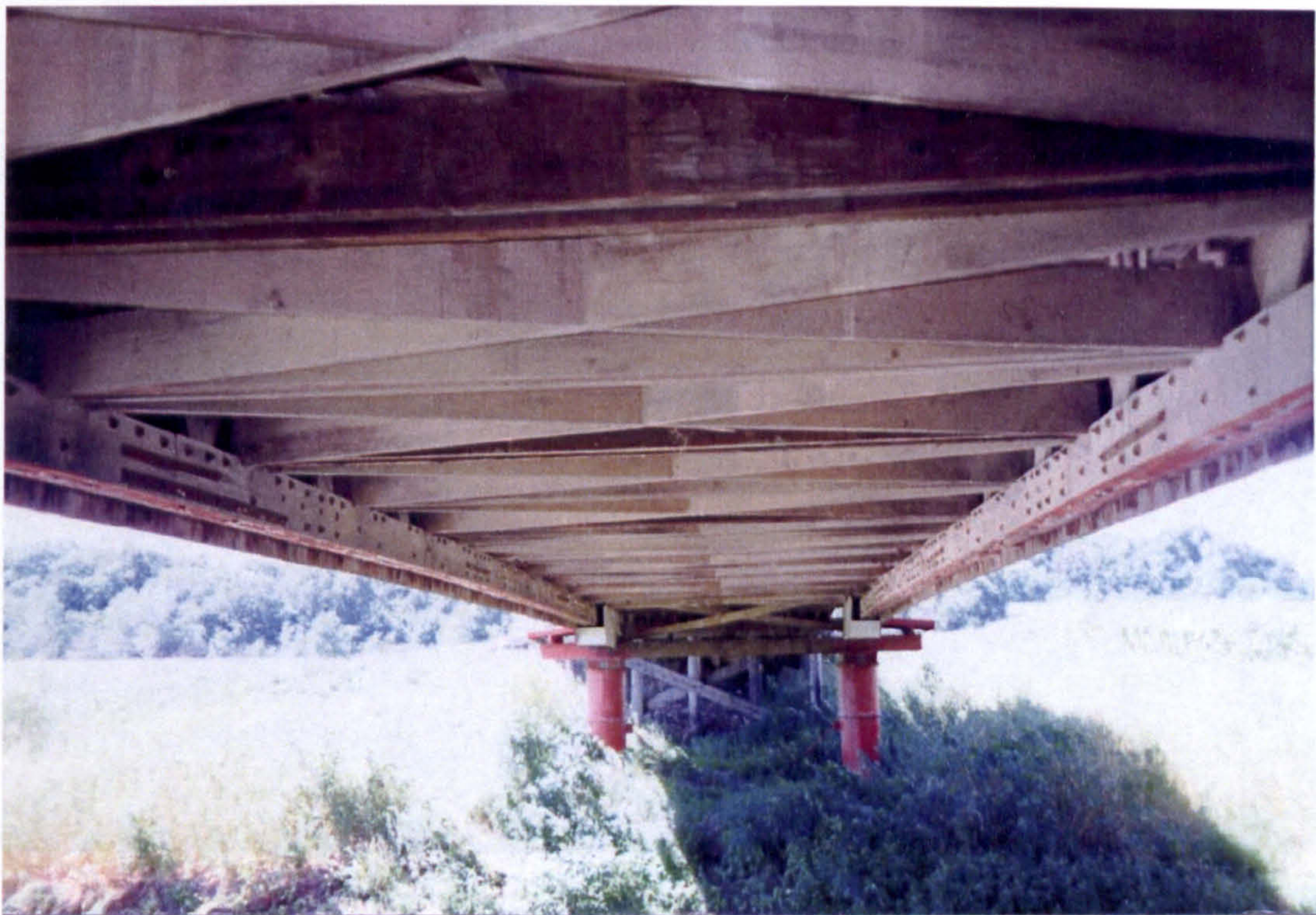
USA – Deck bracing of covered bridge
