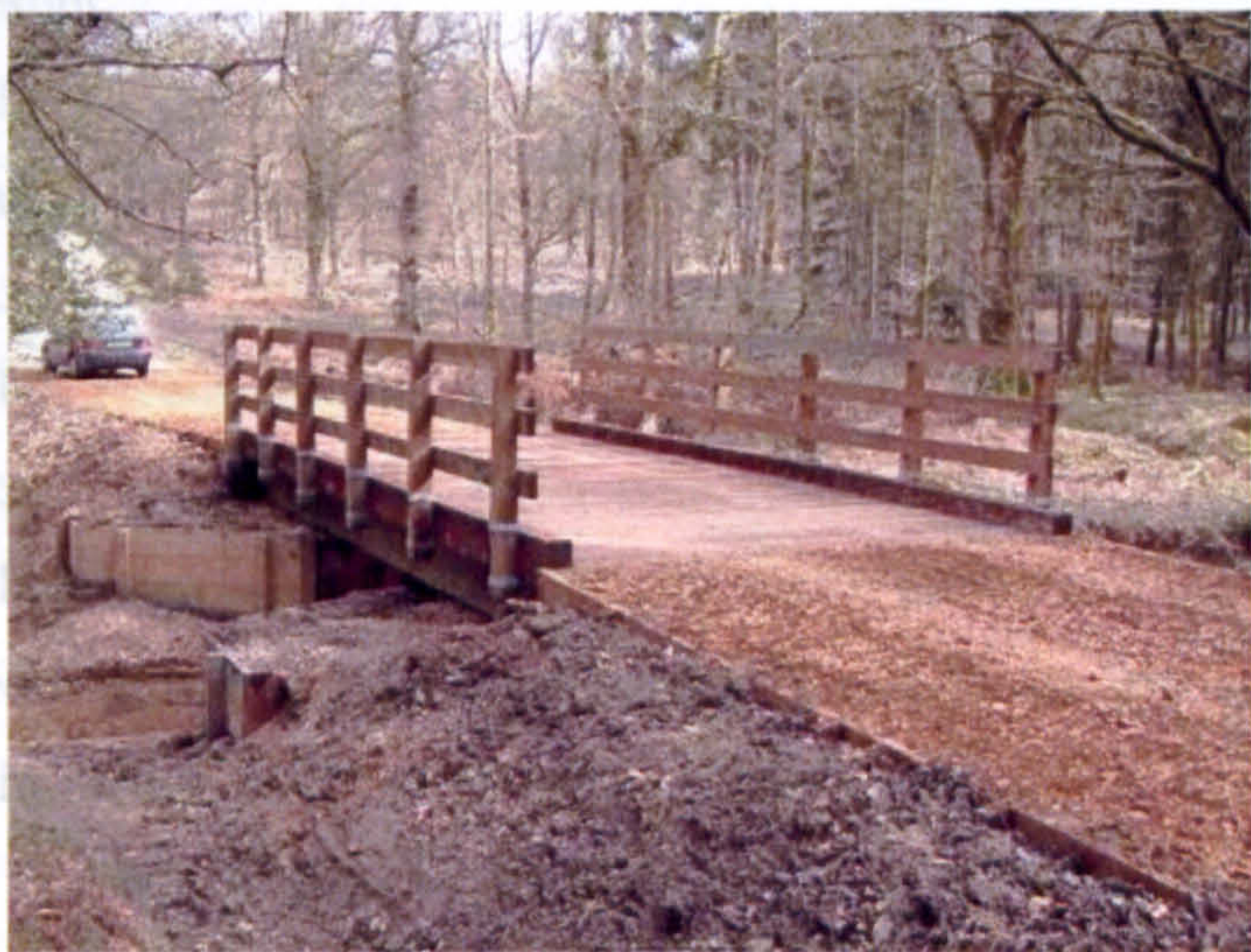
Fig 3.26 - New Forest bridge abutment
