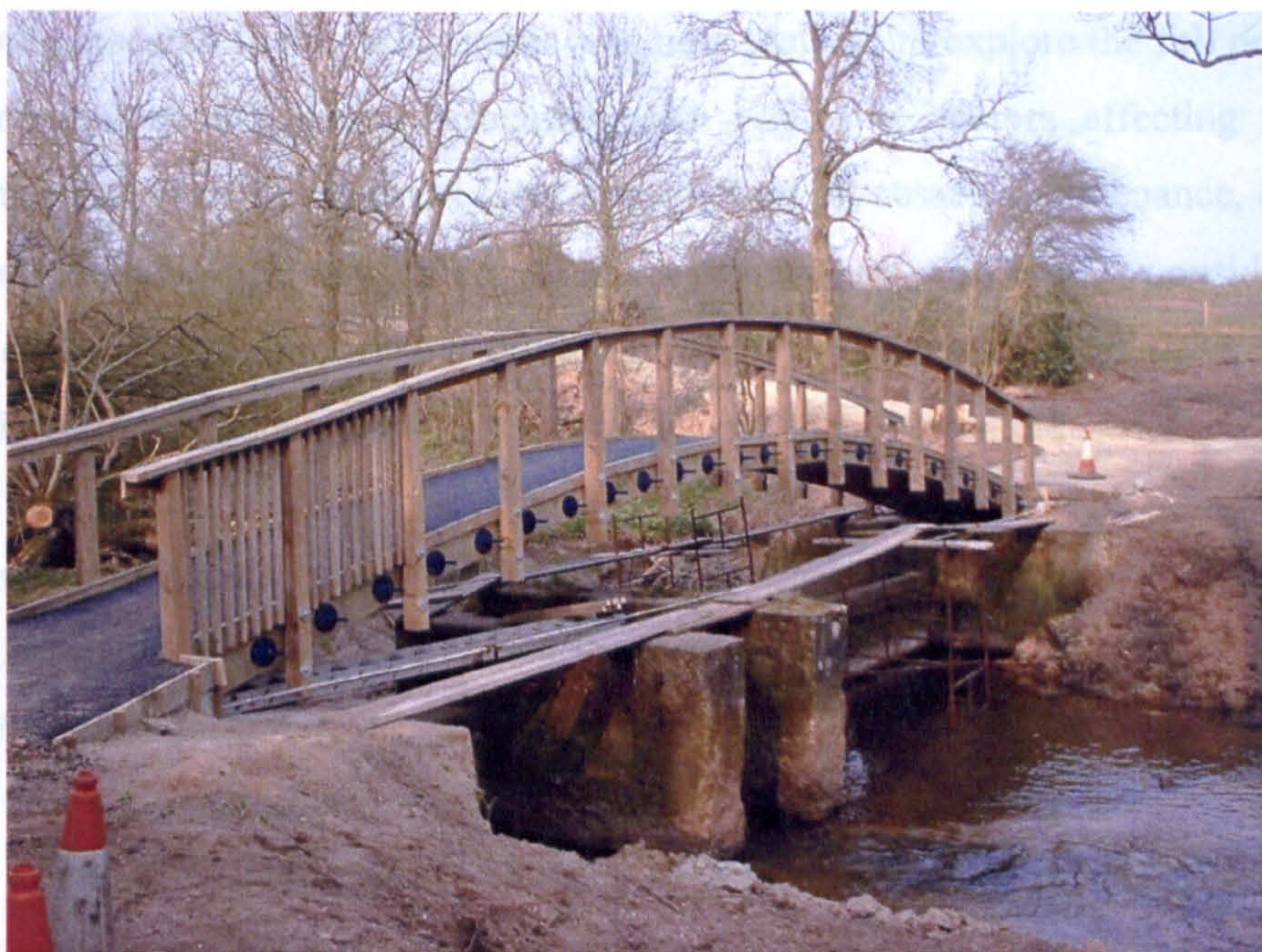
Fig 6.34 -15m span bridge under construction on site
