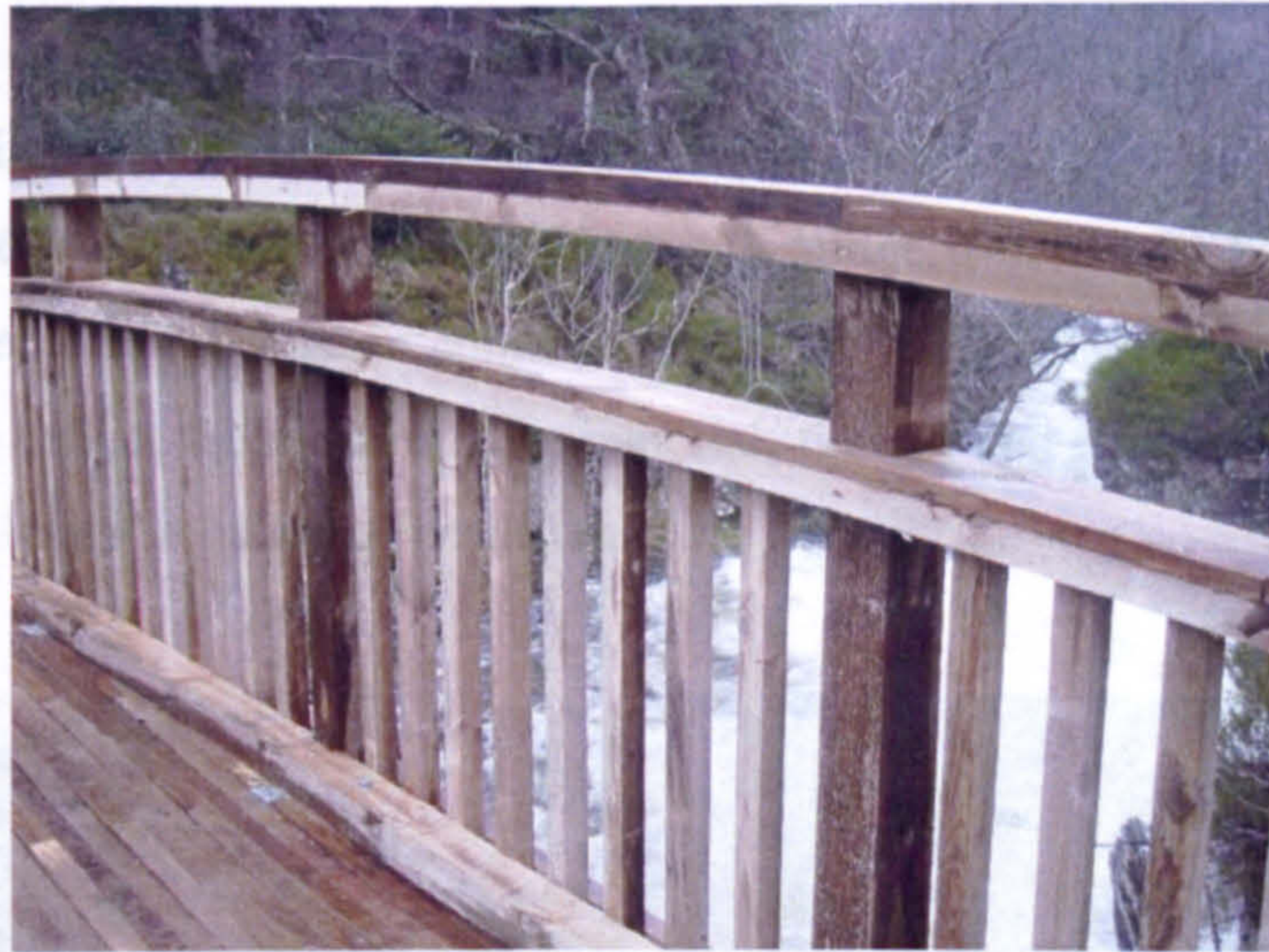
Fig 3.8 - Specialised handrail design - Achray bridge
