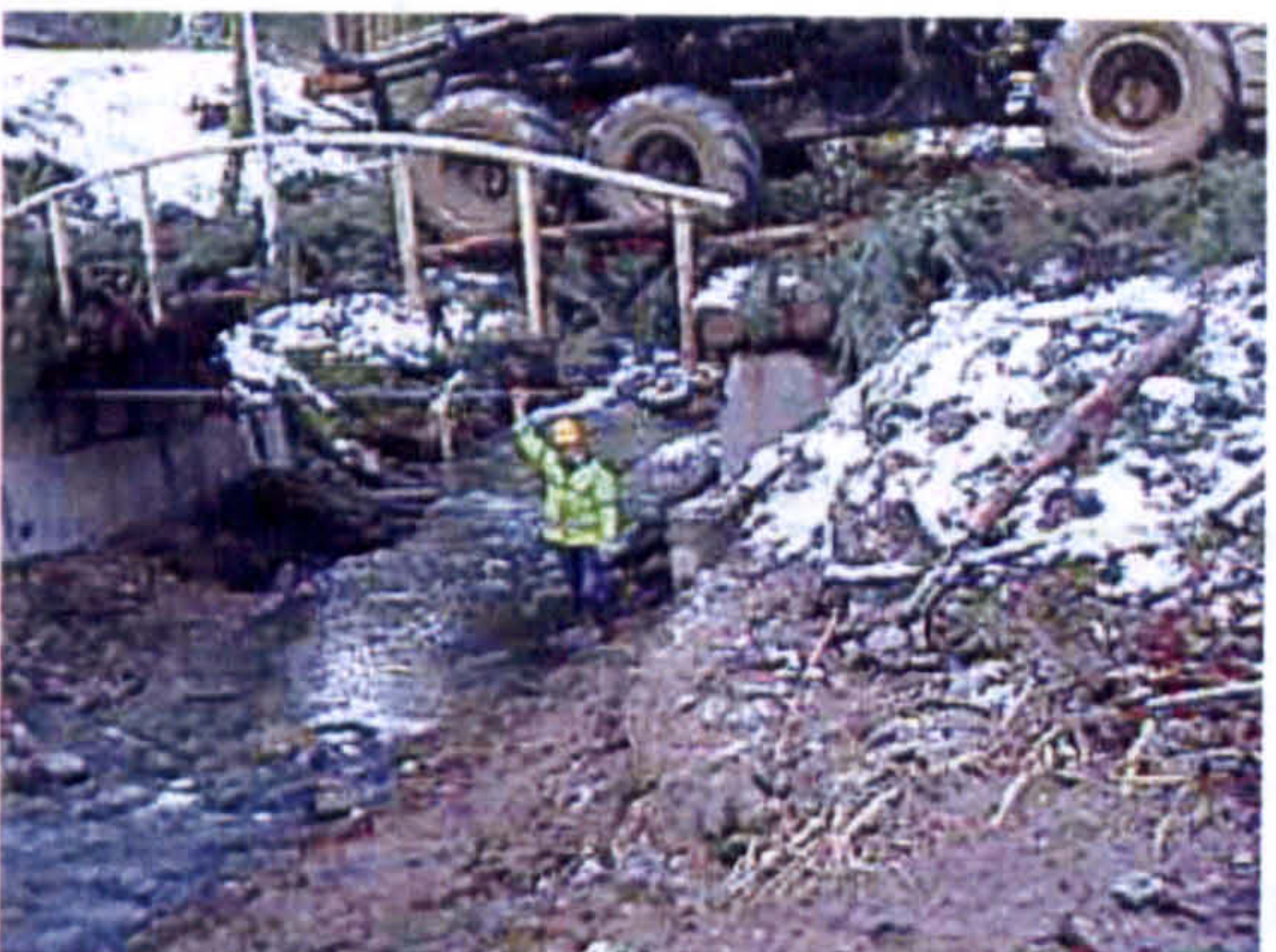
36 tonne harvester crossing on top of a brash mat
