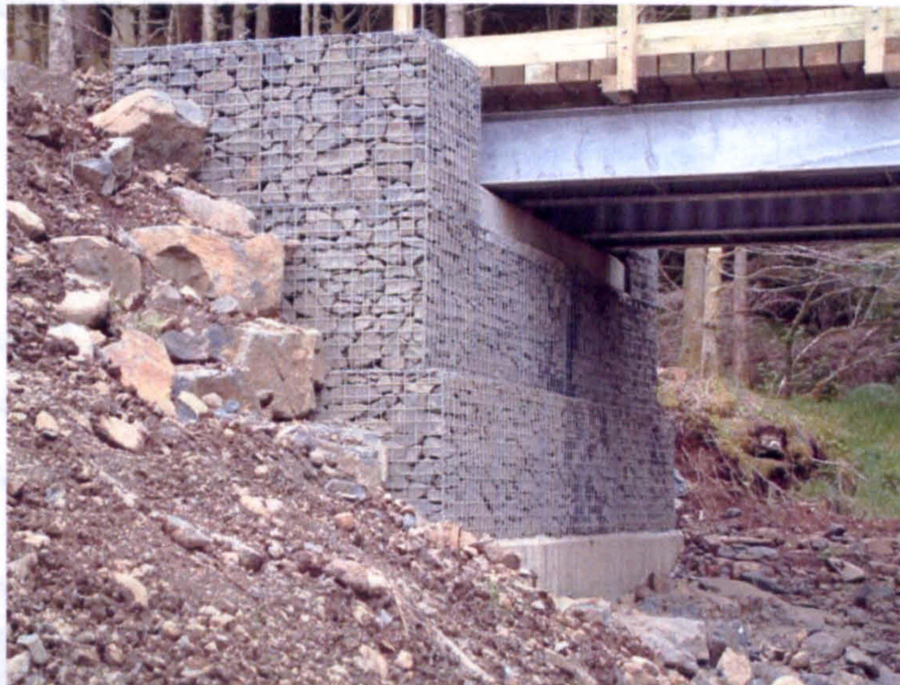
Fig 3.23 - BRC Gabion abutments – sill beam too far forward
