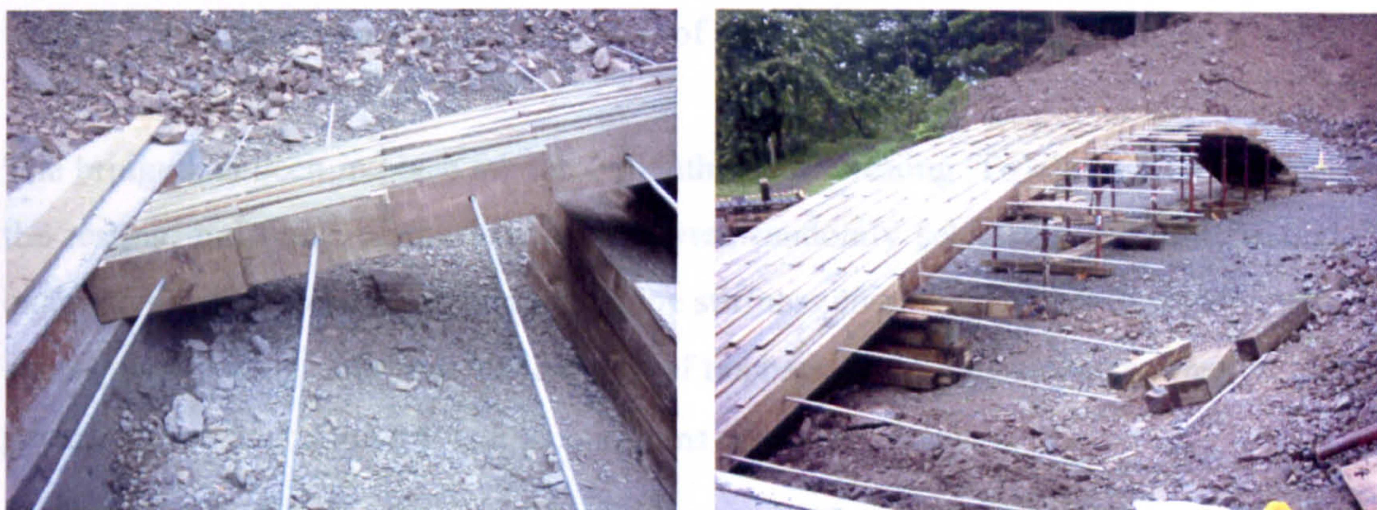
Fig 6.43 – 20m span bridge under construction
