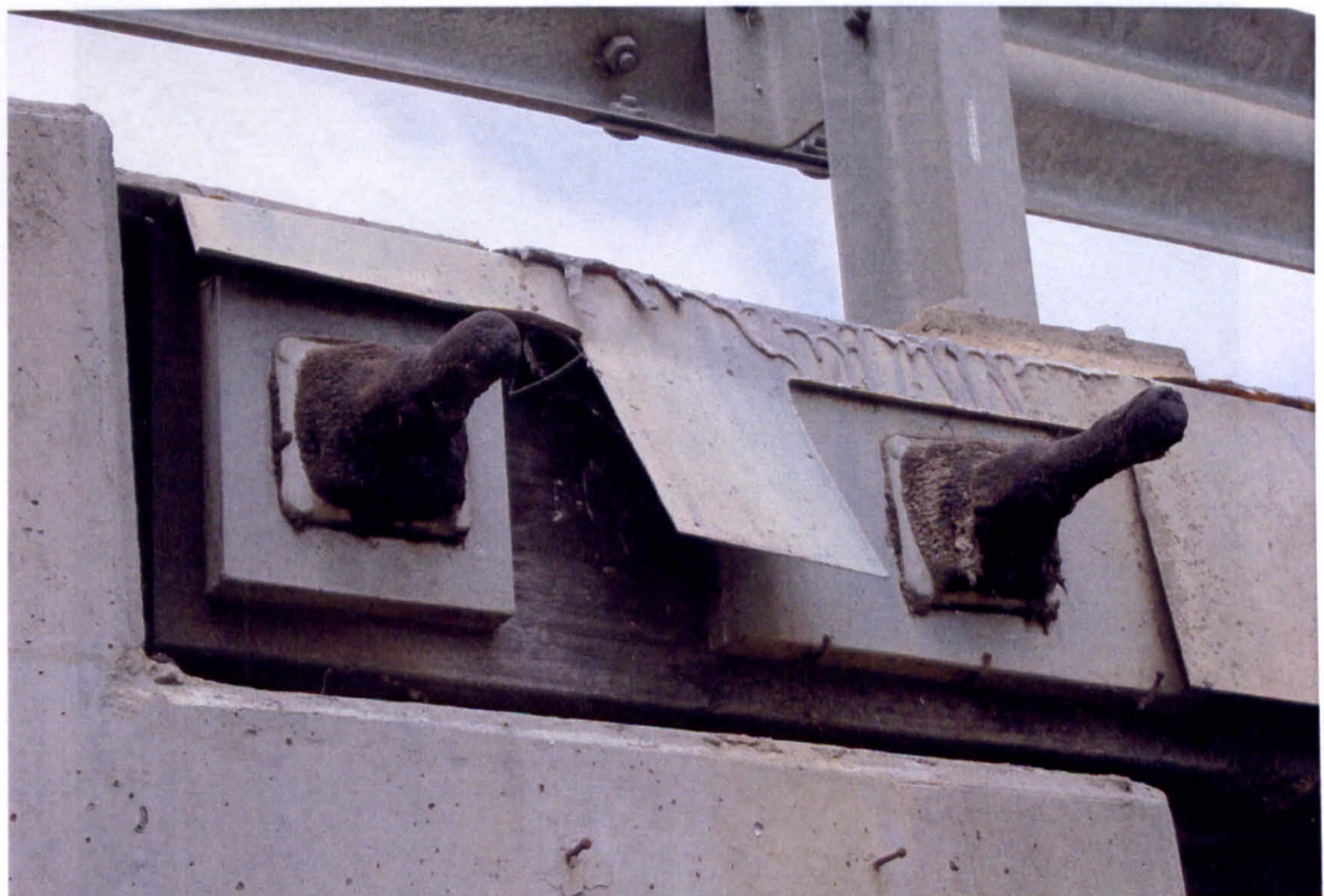
AUS - Metal plates to keep timber dry and tarred stressing bars to prevent corrosion
