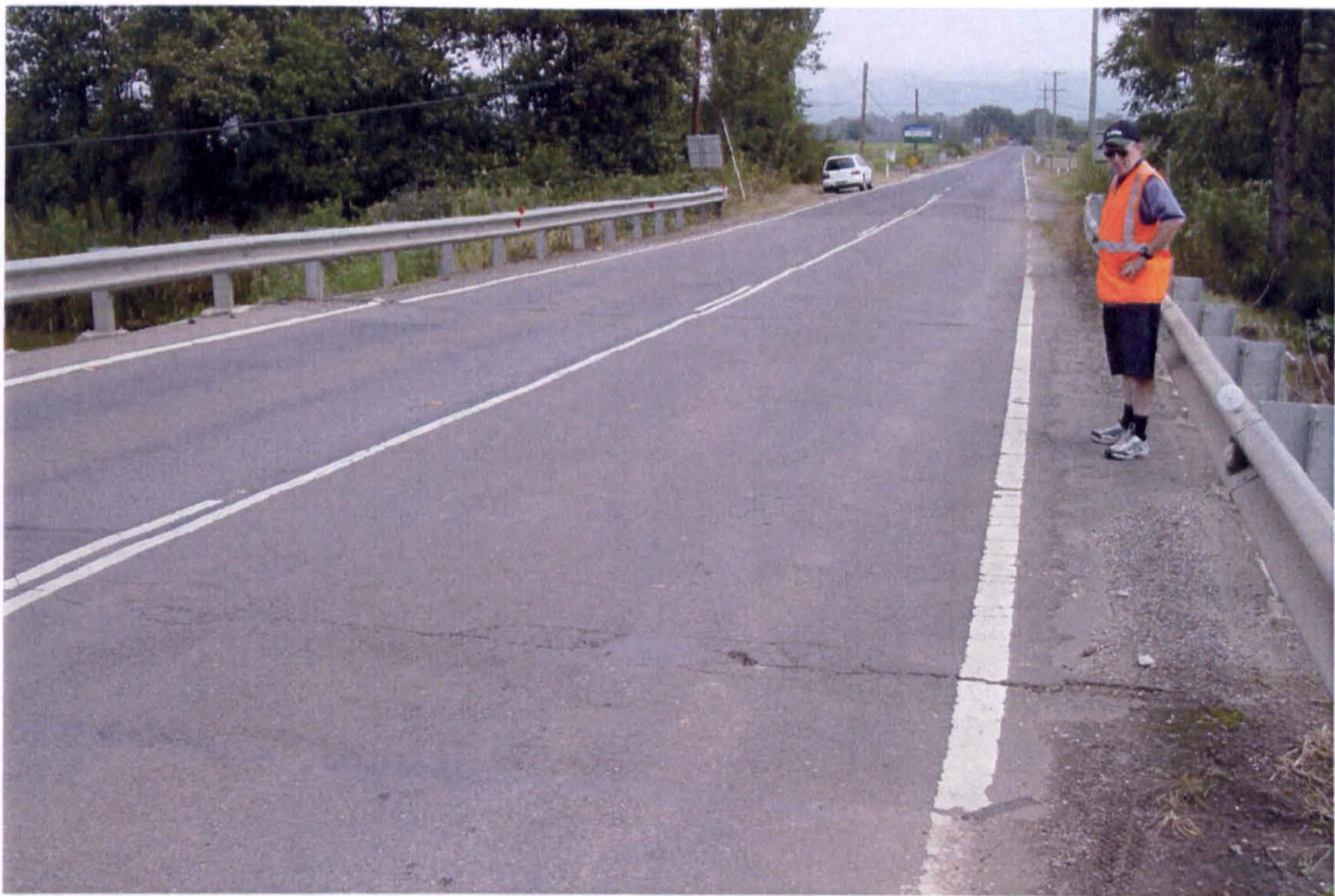
AUS - Cracks at interface between timber deck and abutment resulting from deflection and no designed joint
