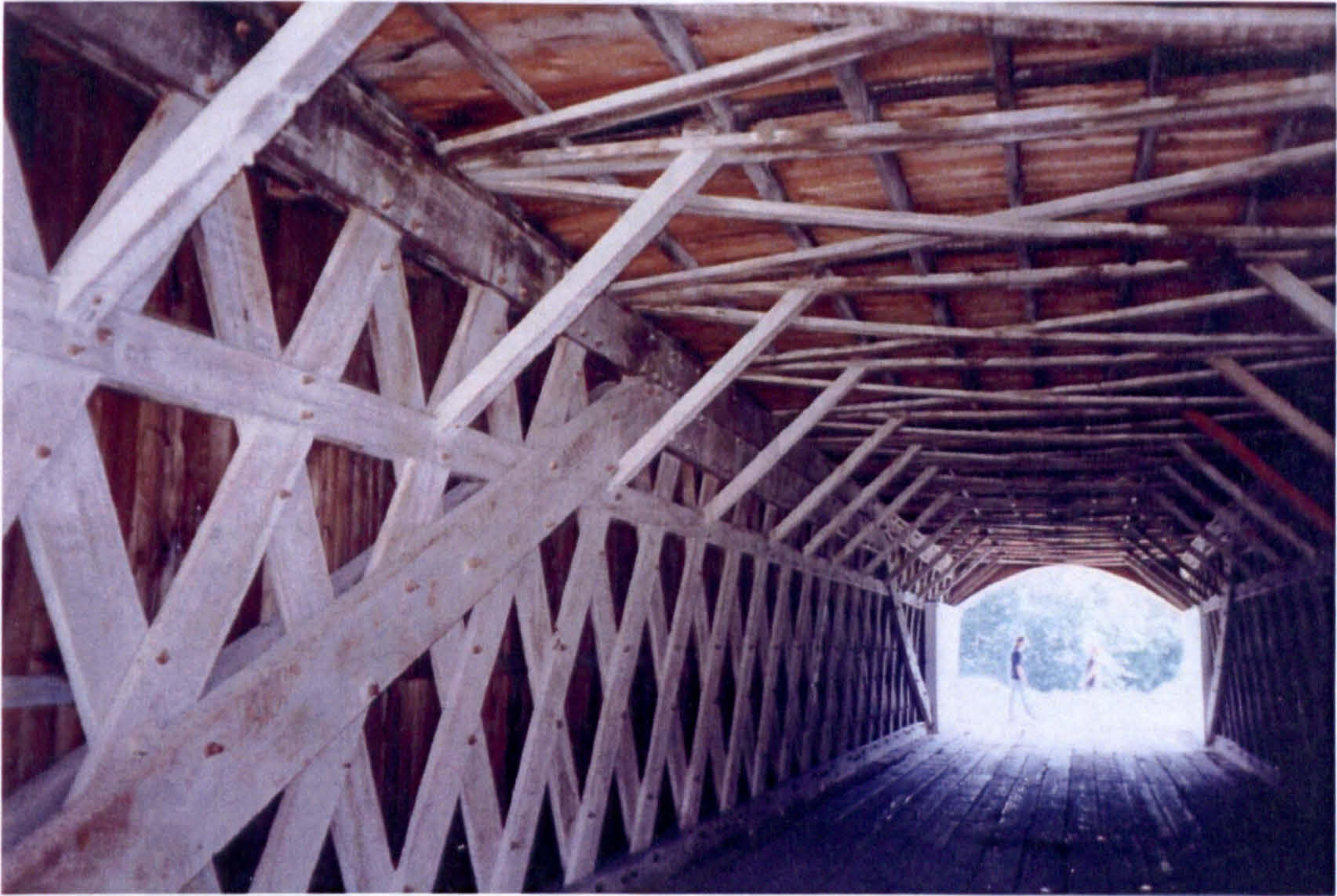
USA – The internal bracing of the Roseman covered bridge in Madison County
