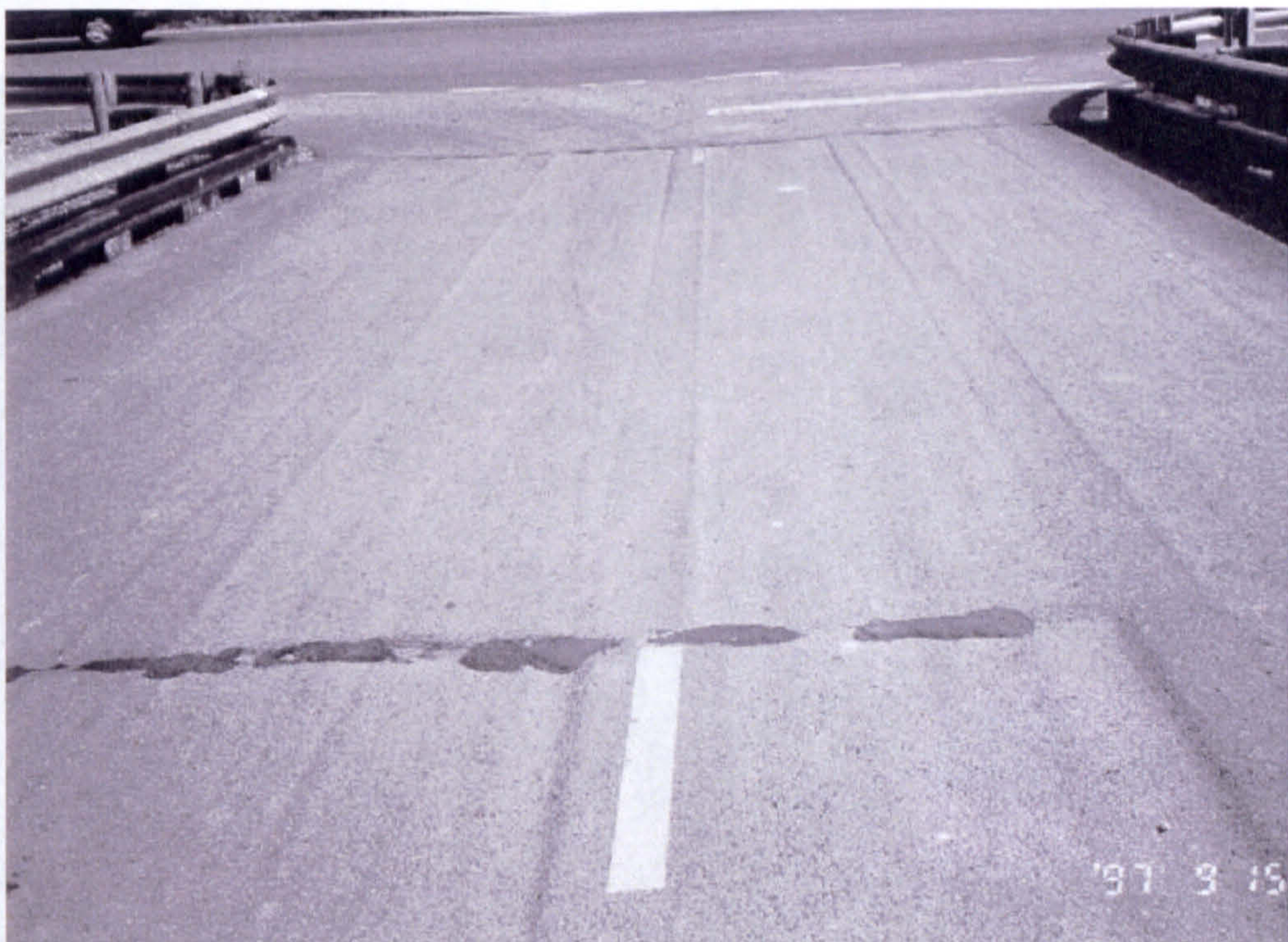
USA – Cracks in asphalt at joints in deck and some slip of laminates
