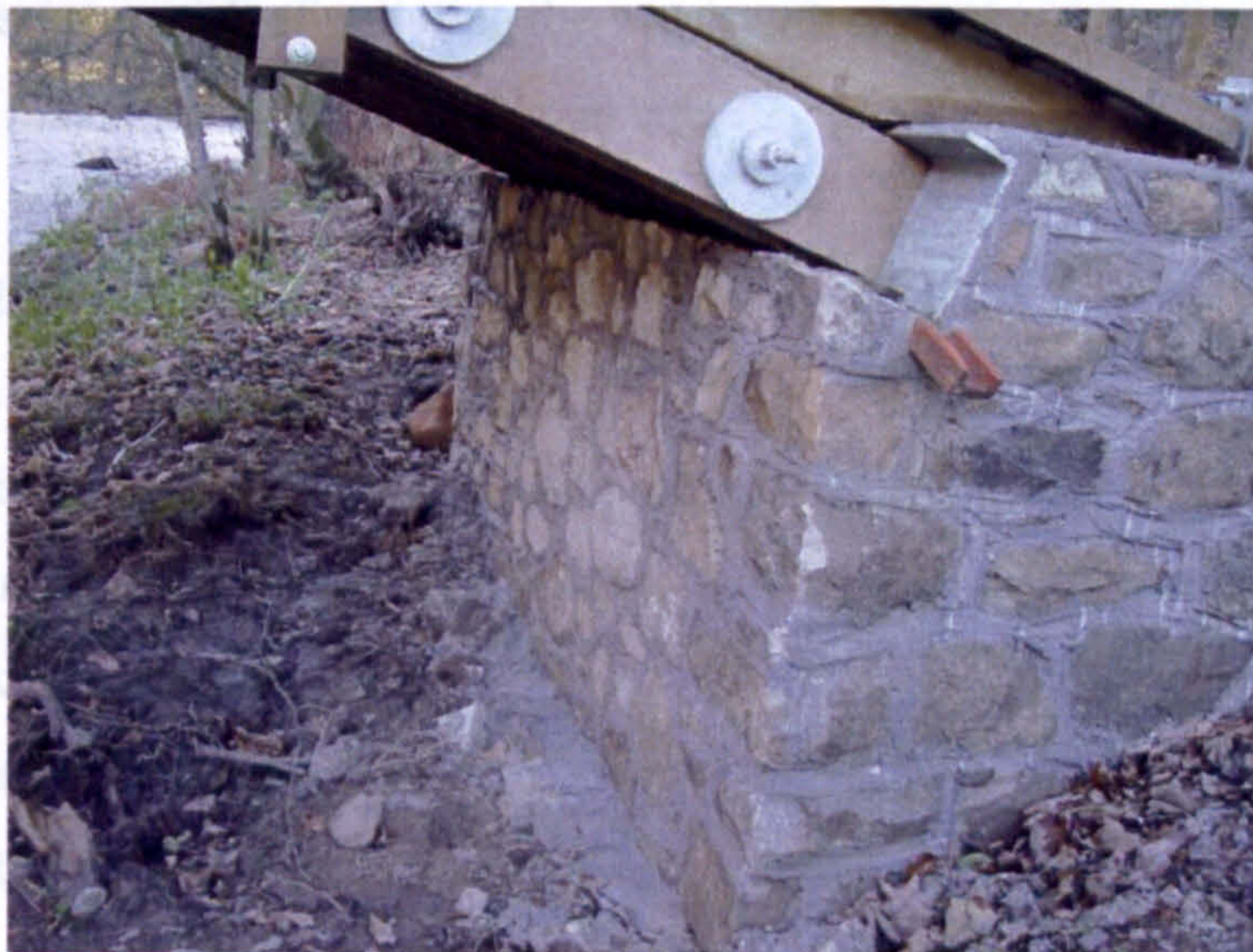
Fig 3.21 - Stone faced concrete abutment – Carribber bridge
