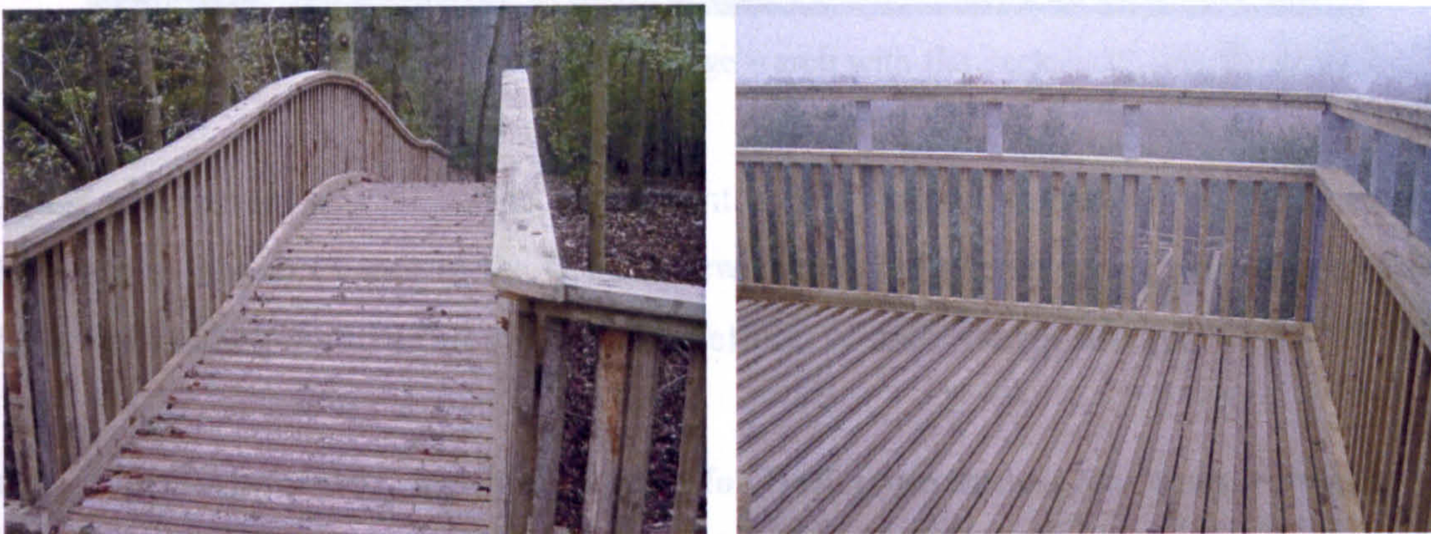
Fig 6.4 – Non slip deck on new bridges at Salcey
