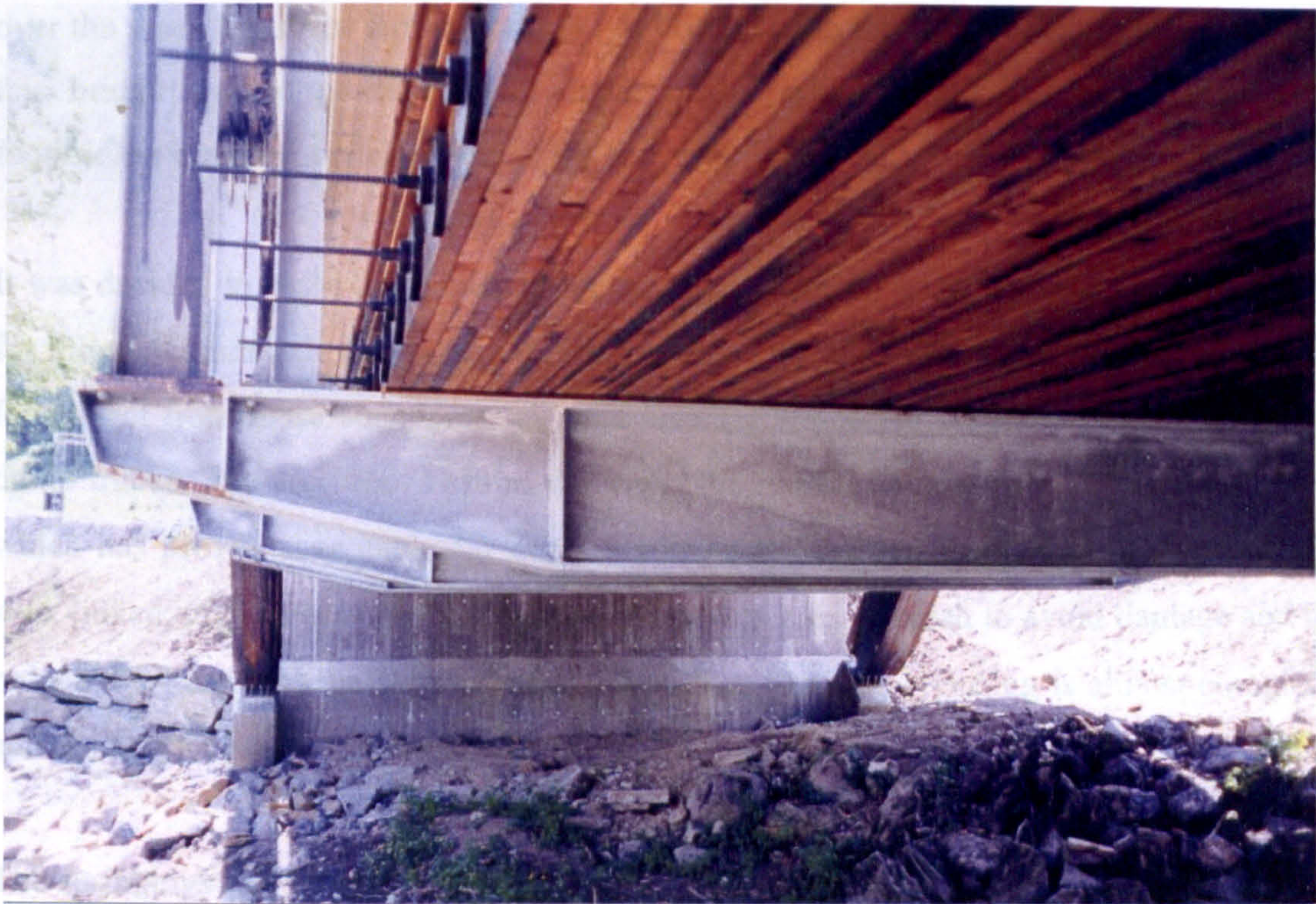
Norway – SLT deck supported by steel cradle beams
