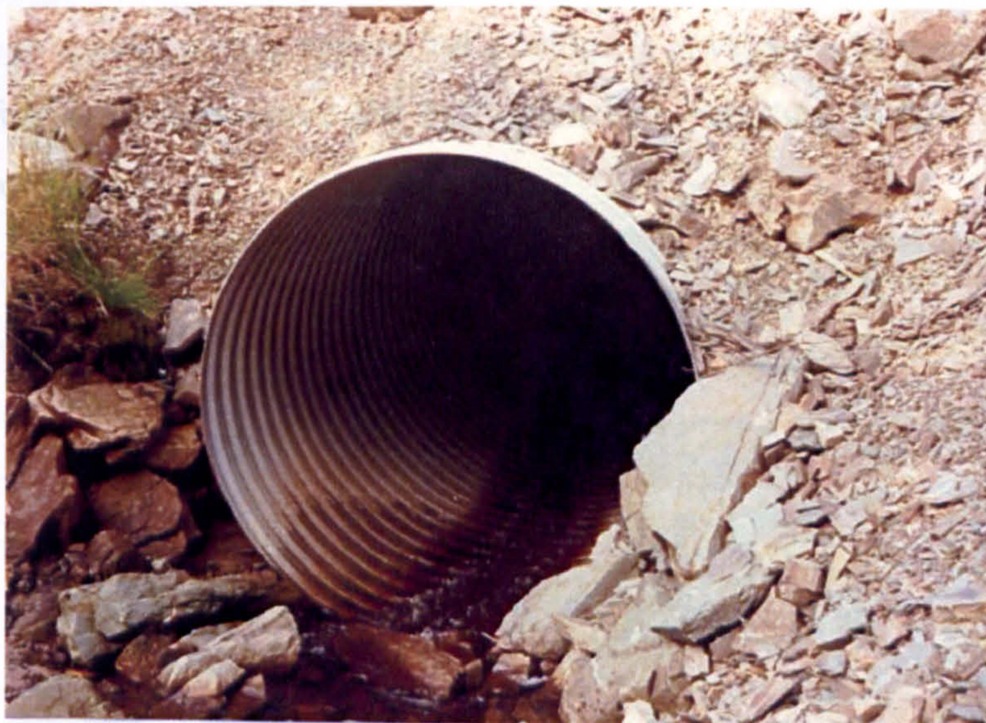
Fig 3.16 - Corrugated steel culvert – corroding and too high above the stream bed
