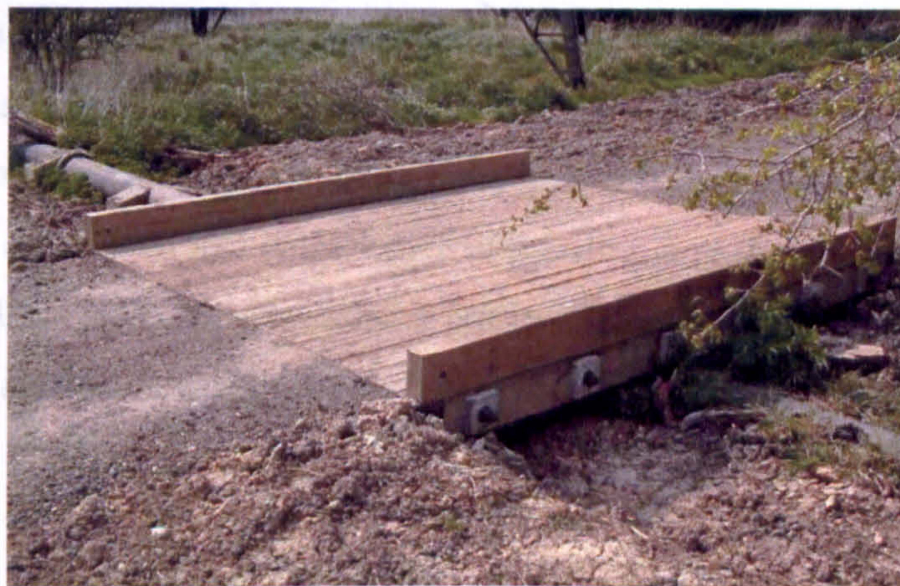
Fig 6.1 - First SLT bridge – Macalloy bars
