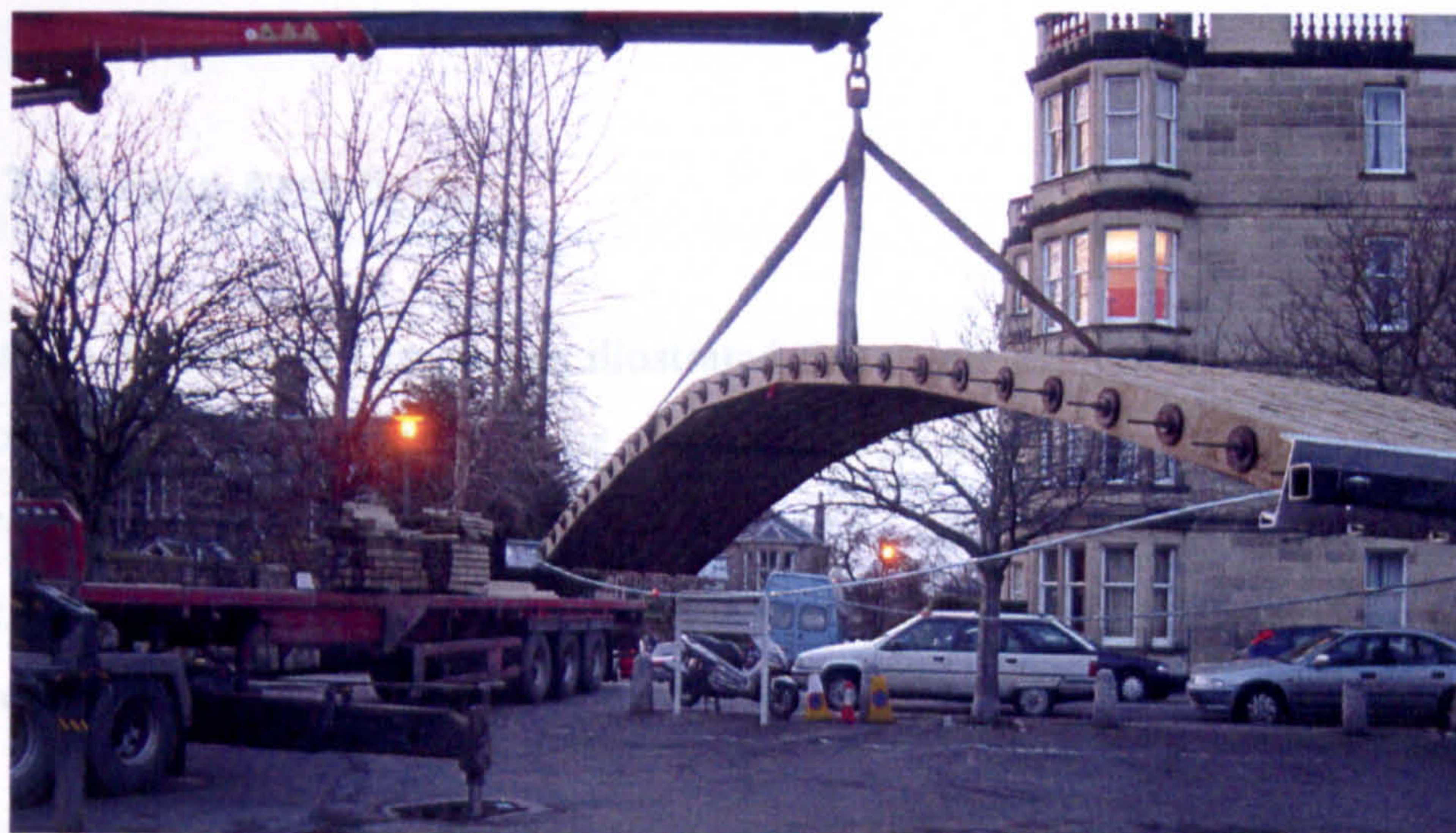
Fig 6.33 – Loading 15m span onto lorry
