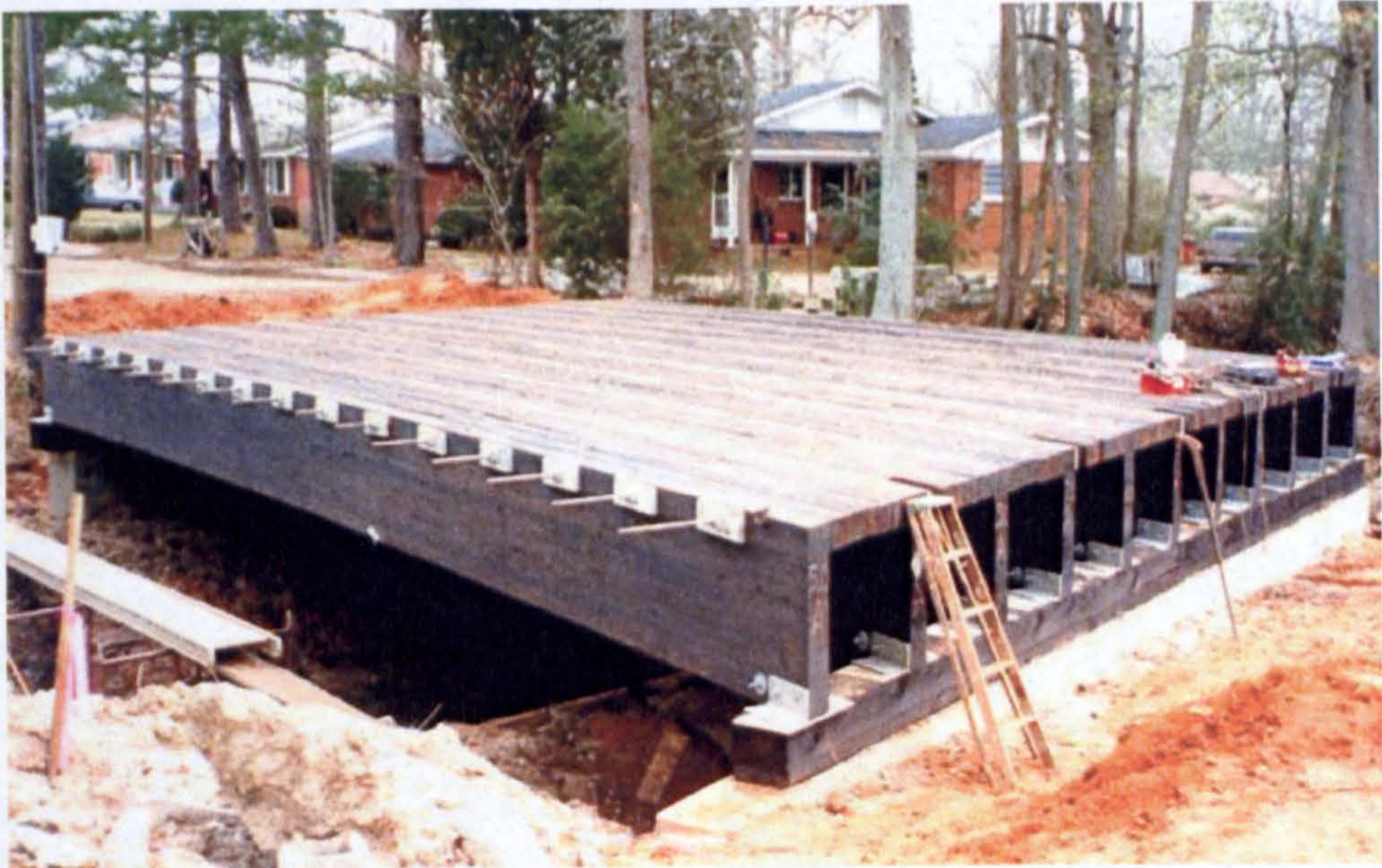
USA – Typical “T” beam deck
