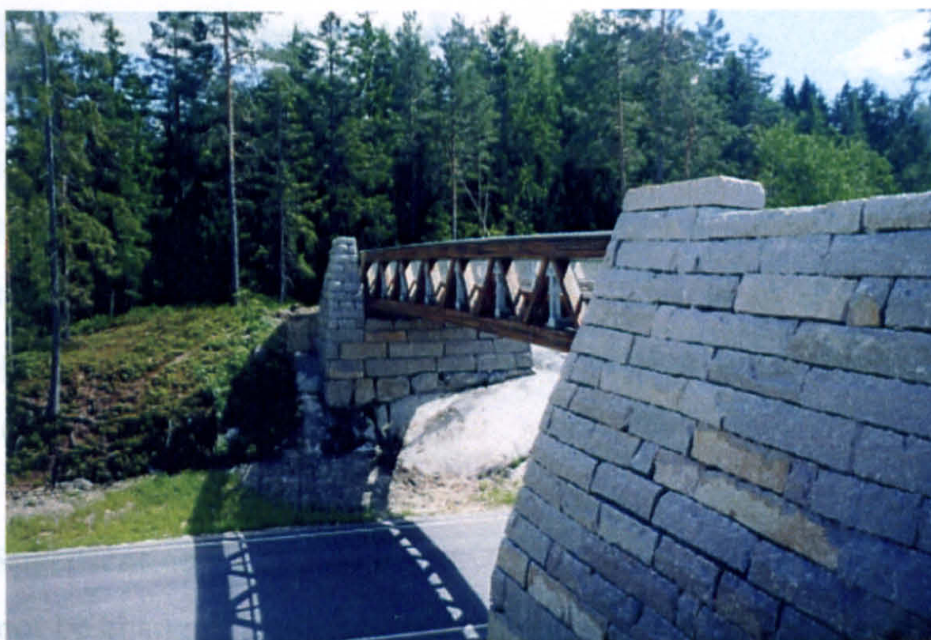
Fig 3.4 - Timber truss and SLT deck bridge over motorway near Oslo, Norway
