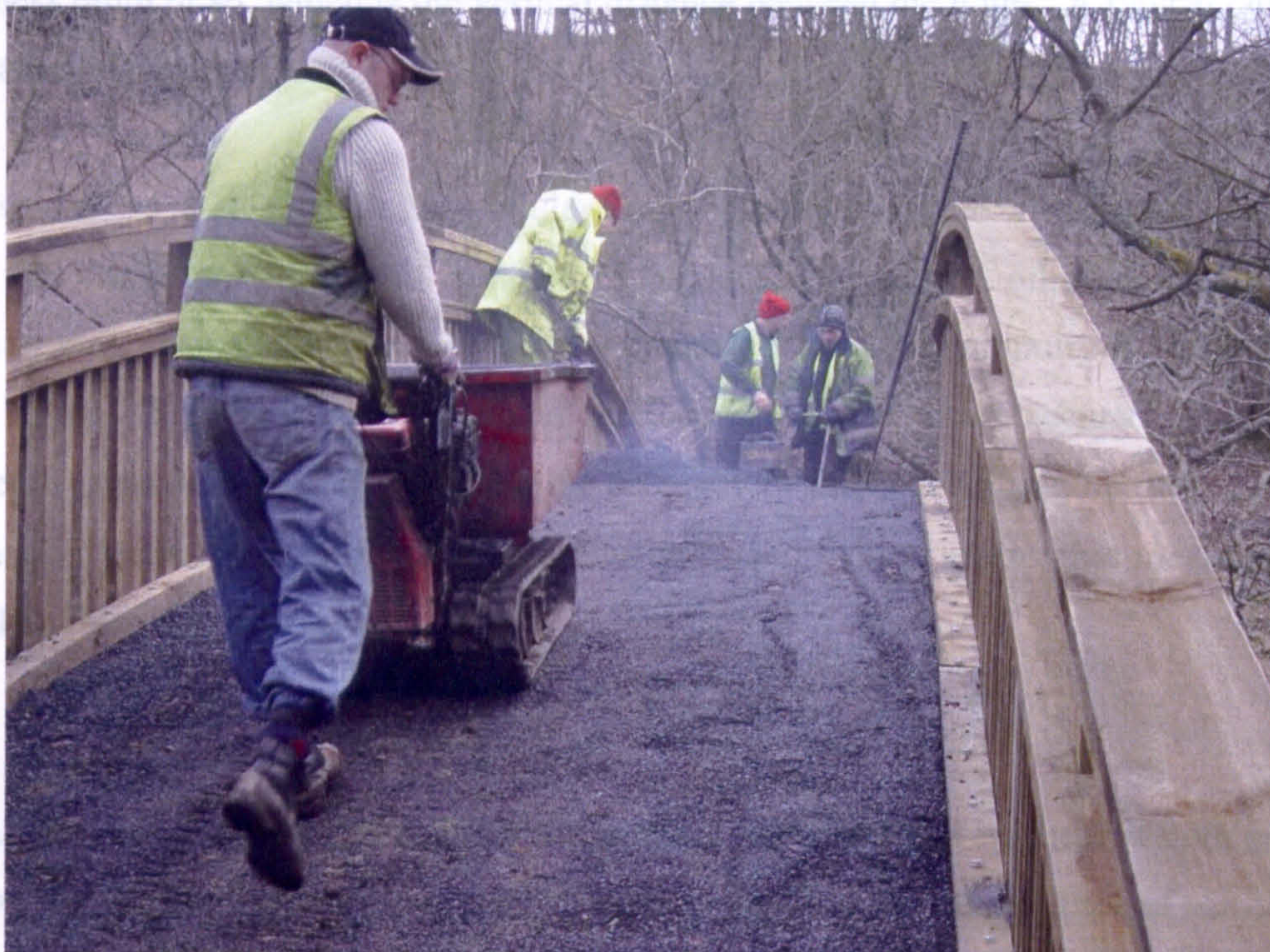
Fig 6.15- Application of Bitmac to bridge deck
