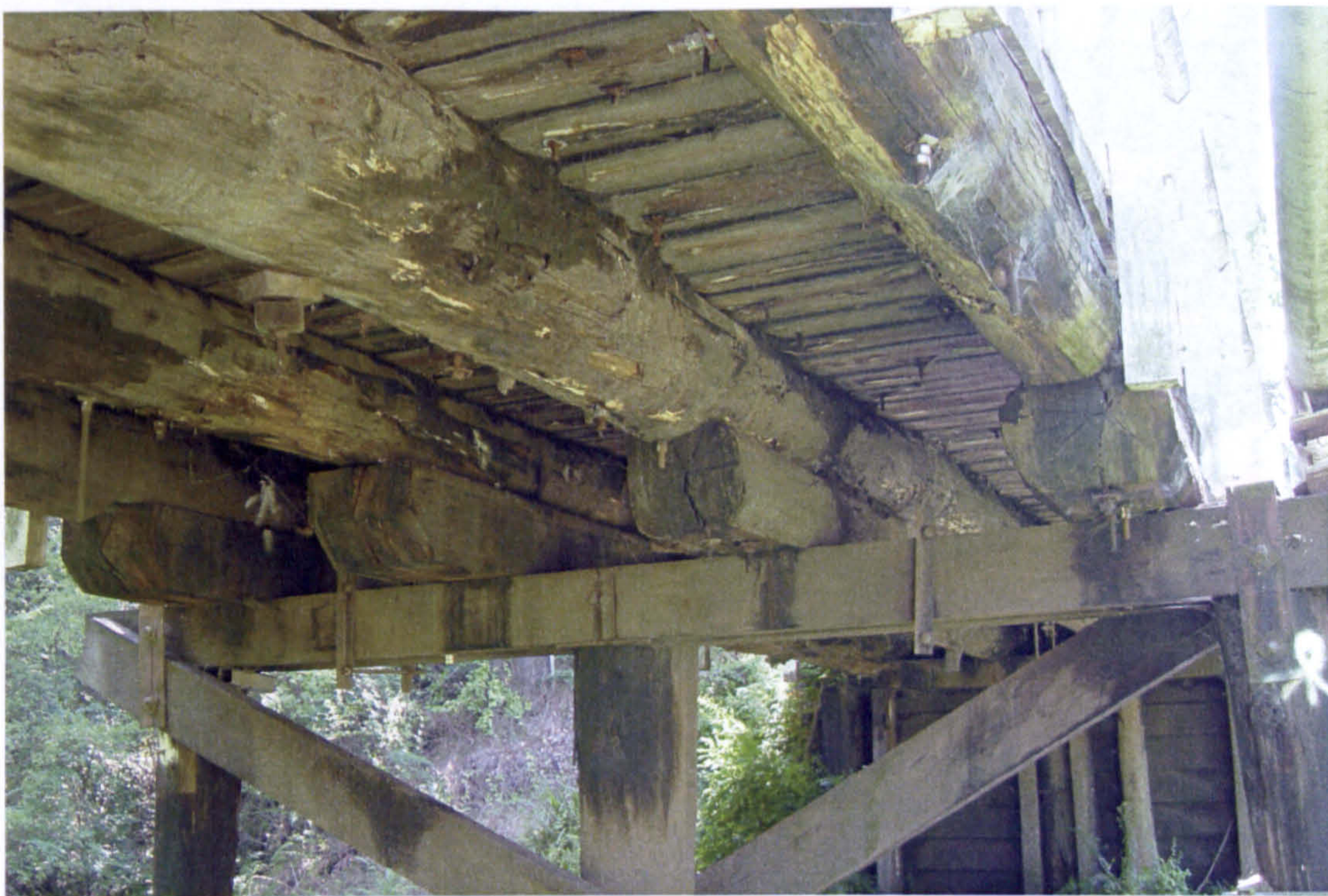
AUS - Typical bridge deck being replaced by SLT deck
