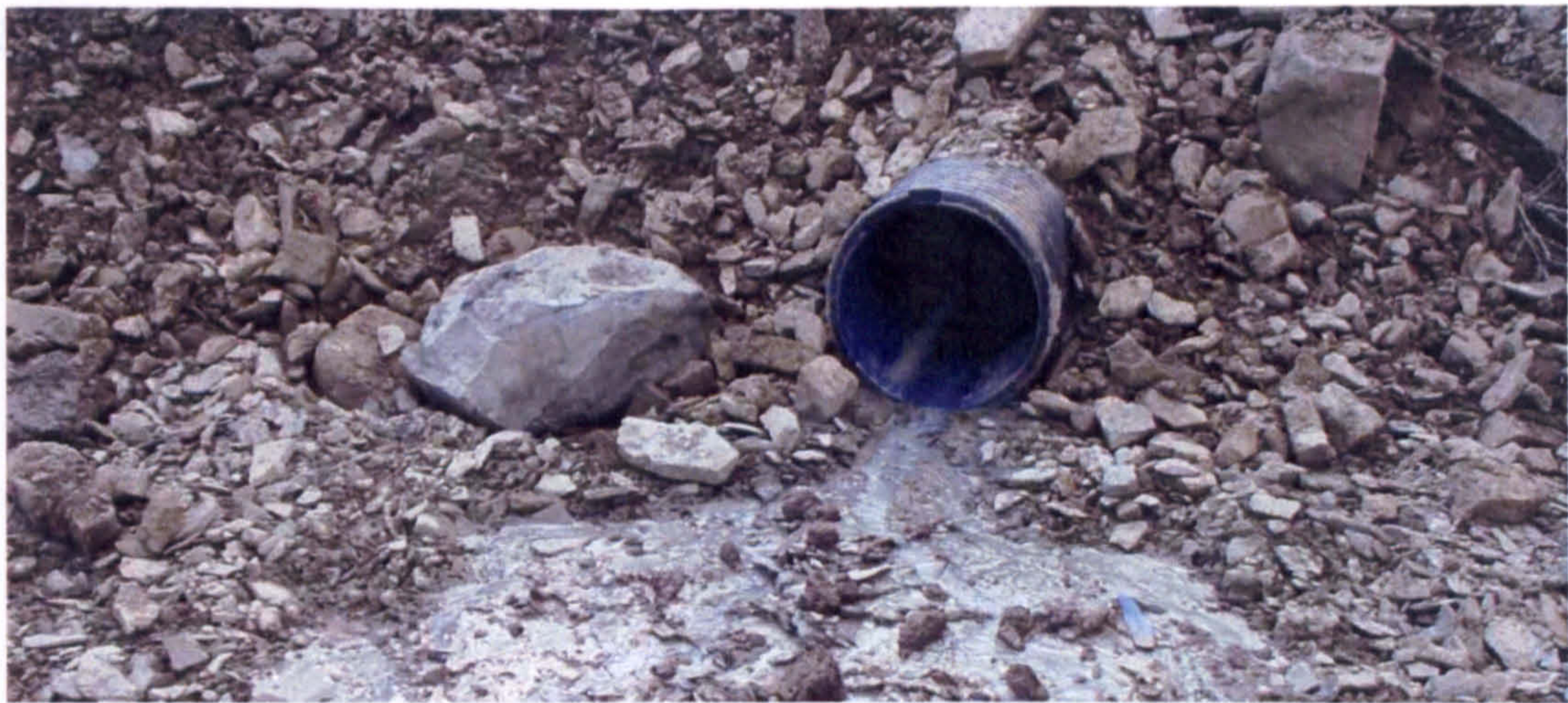
Fig 3.17 - Twin walled plastic culvert
