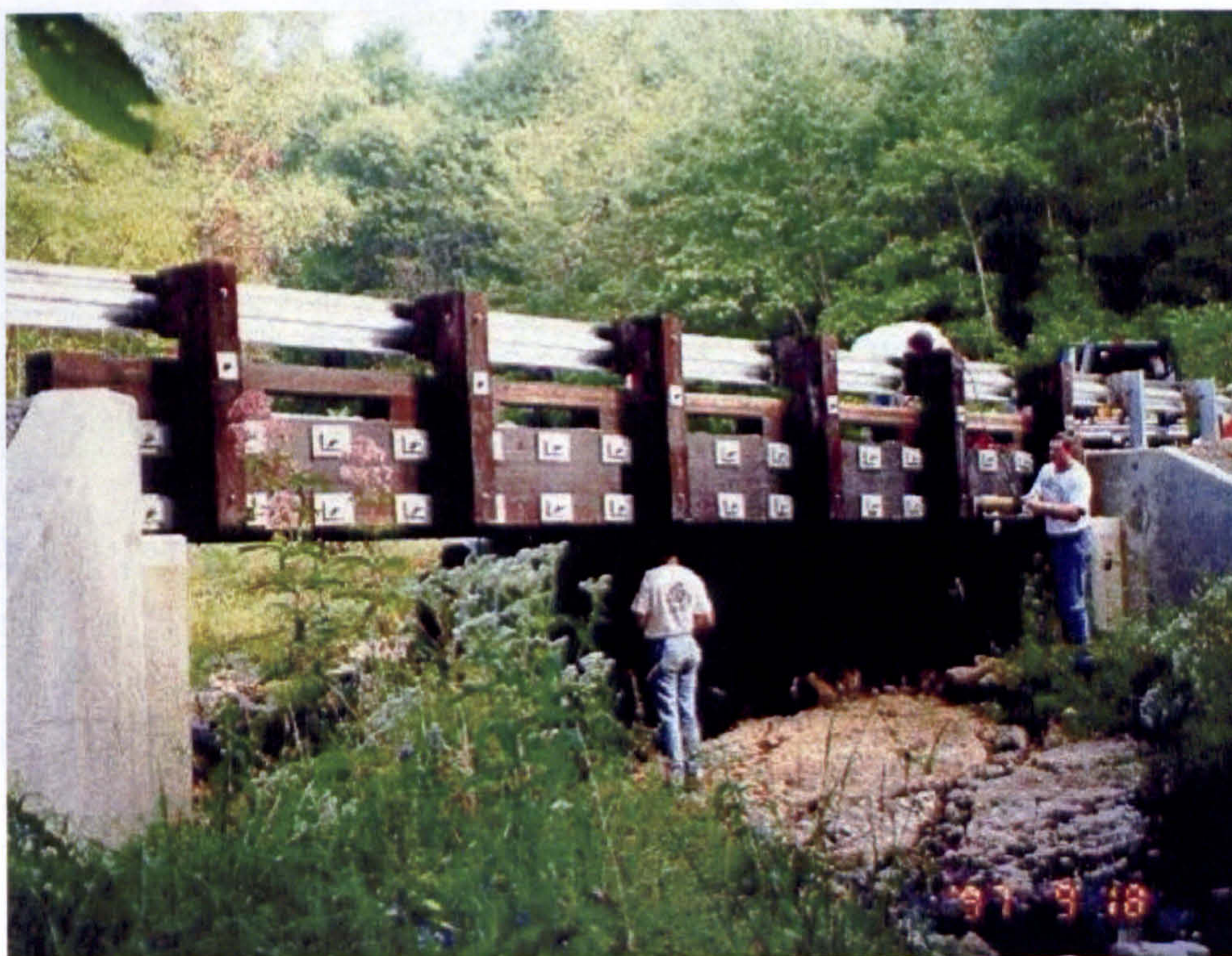
USA – Typical cellular deck for full highway loading
