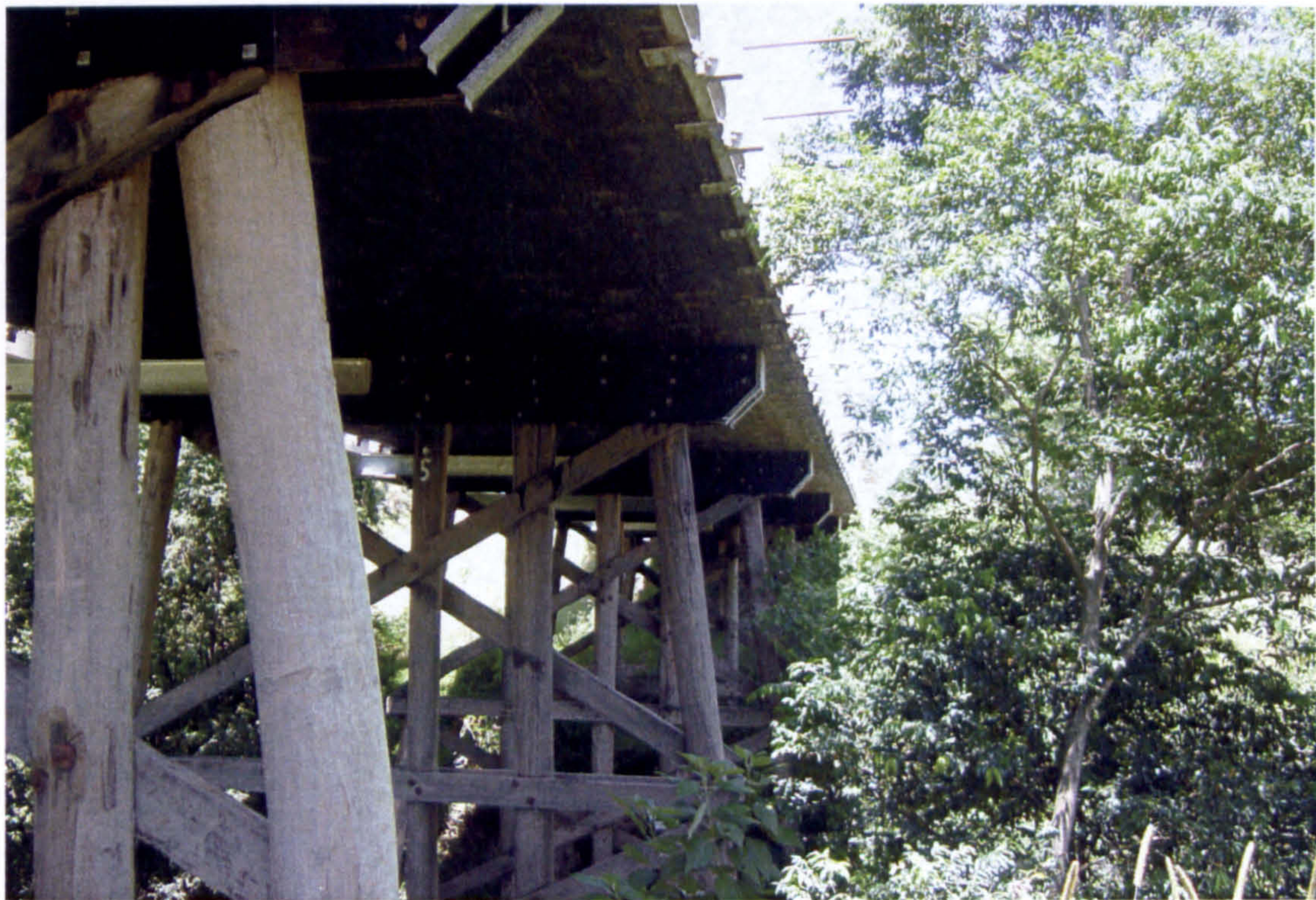
AUS - AUS - Typical round timber braced piers supporting SLT deck
