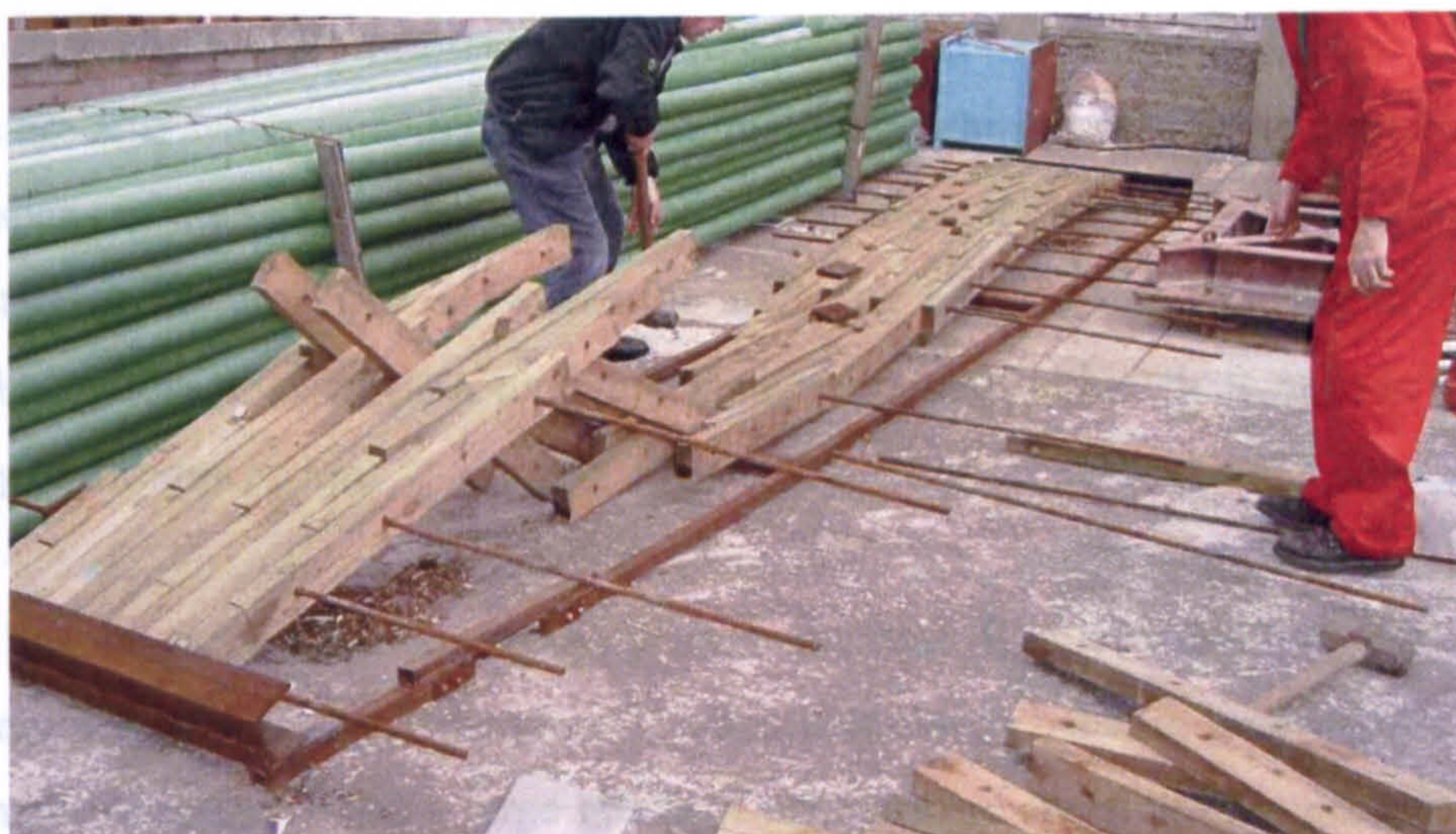
Fig 5.17 - Dismantling 6m trial arch
