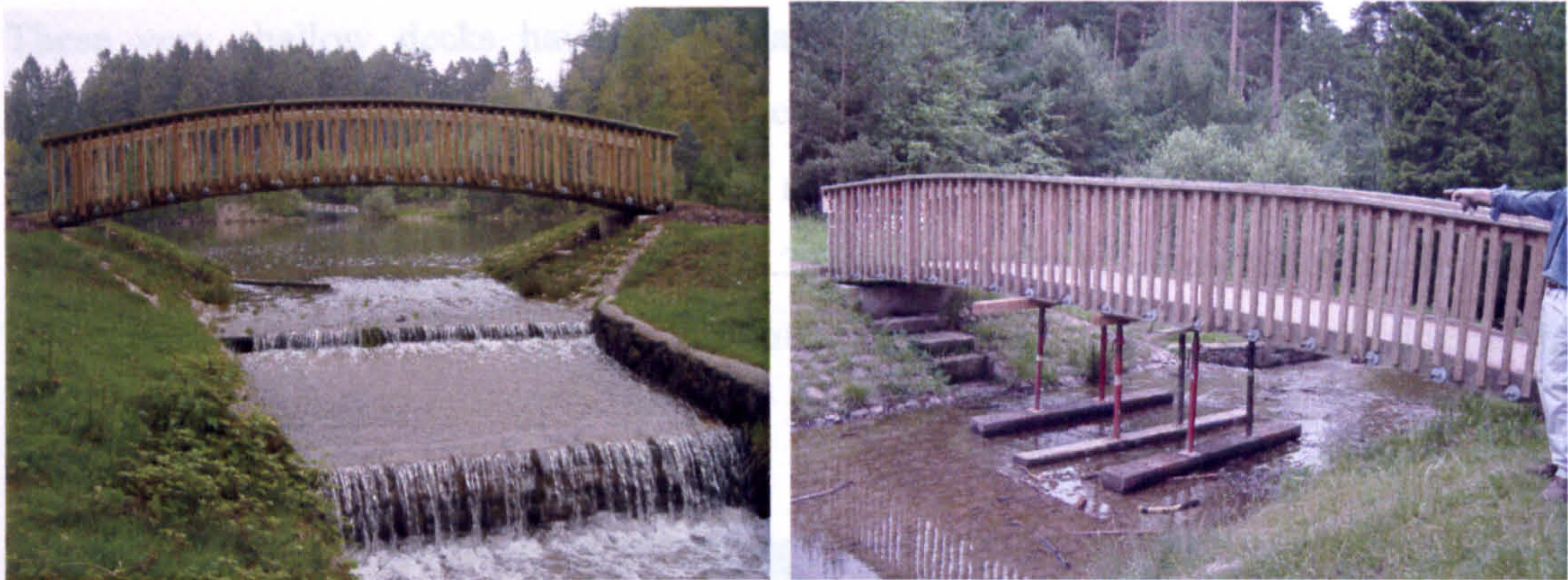
Fig 5.25 – Mallard Pike, Forest of Dean - completed too flat and collapsed
