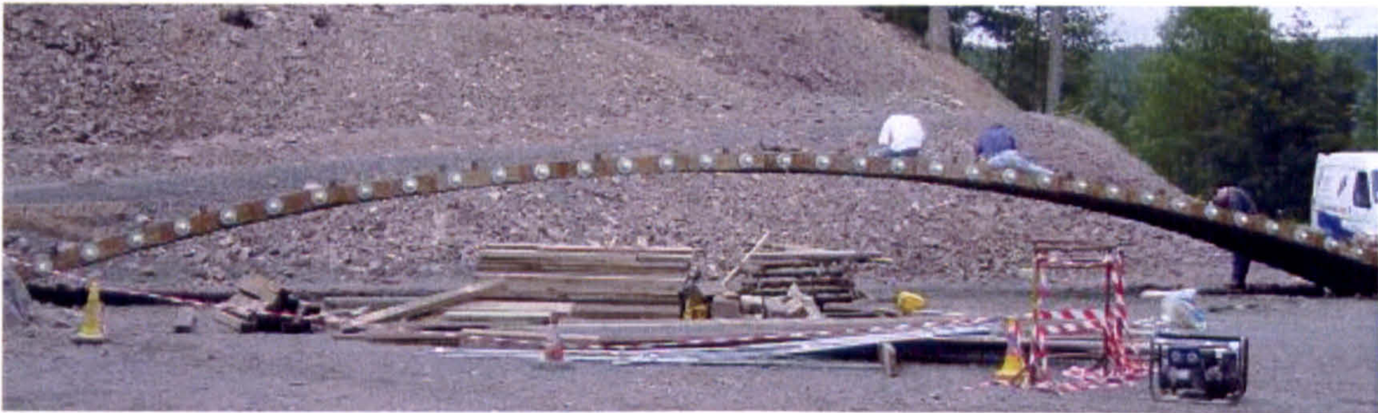
Fig 5.18 - 20m Test bridge at Glentress during construction – span/depth 1/100
