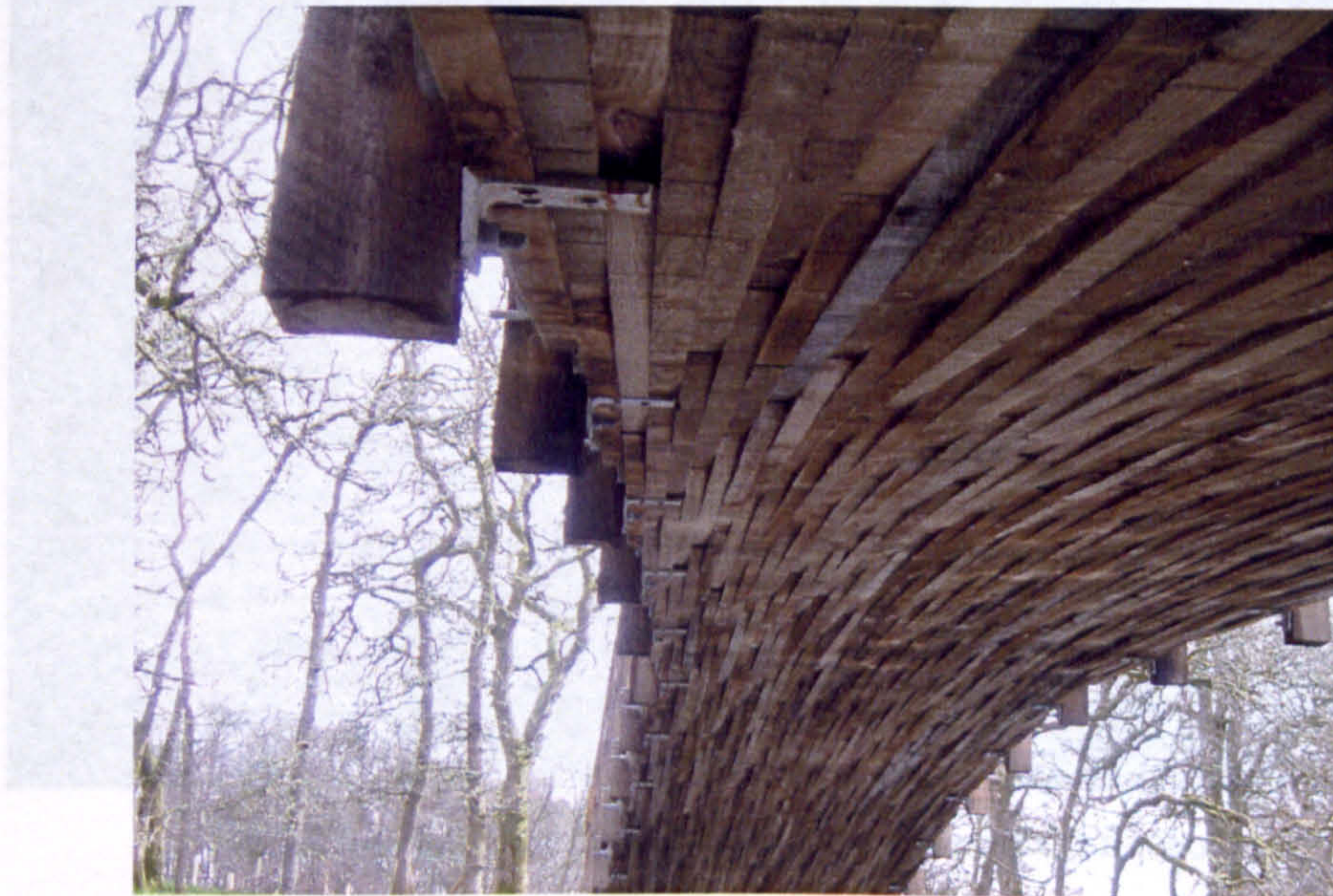
Fig 5.26– Brackets for handrail posts
