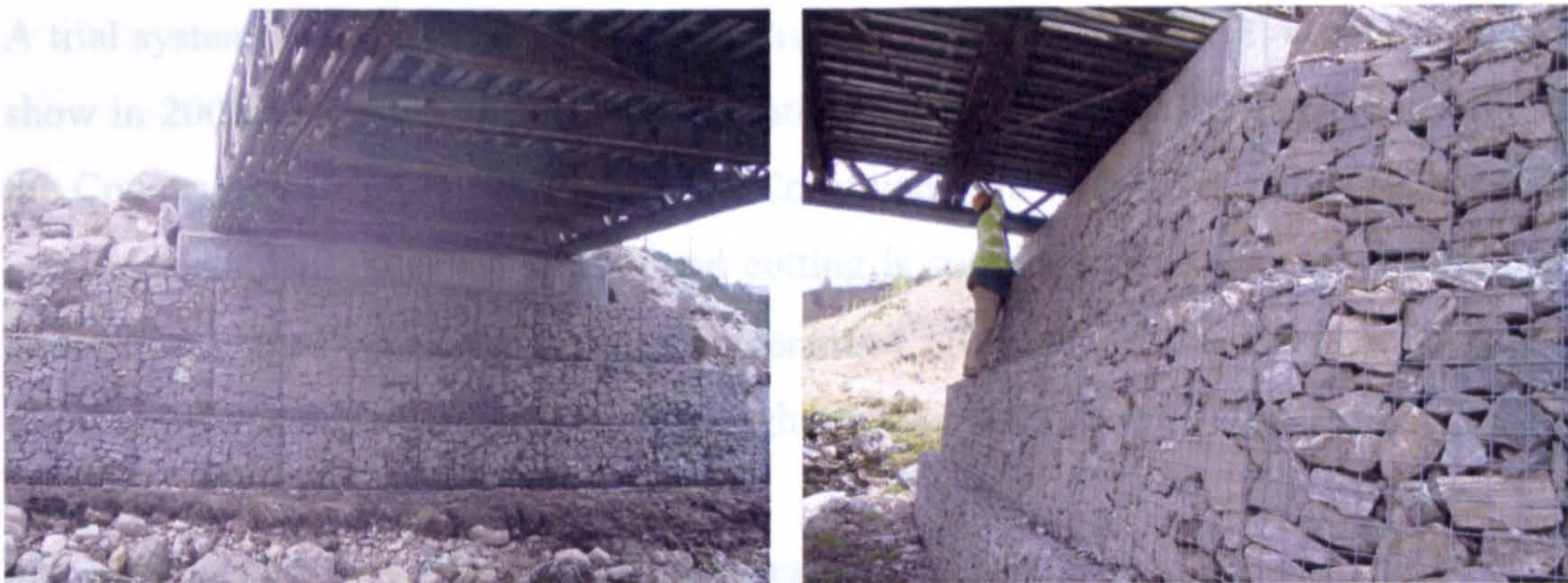
Fig 3.25 - Gabion abutment face to a geotextile abutment – Farr Wind Farm
