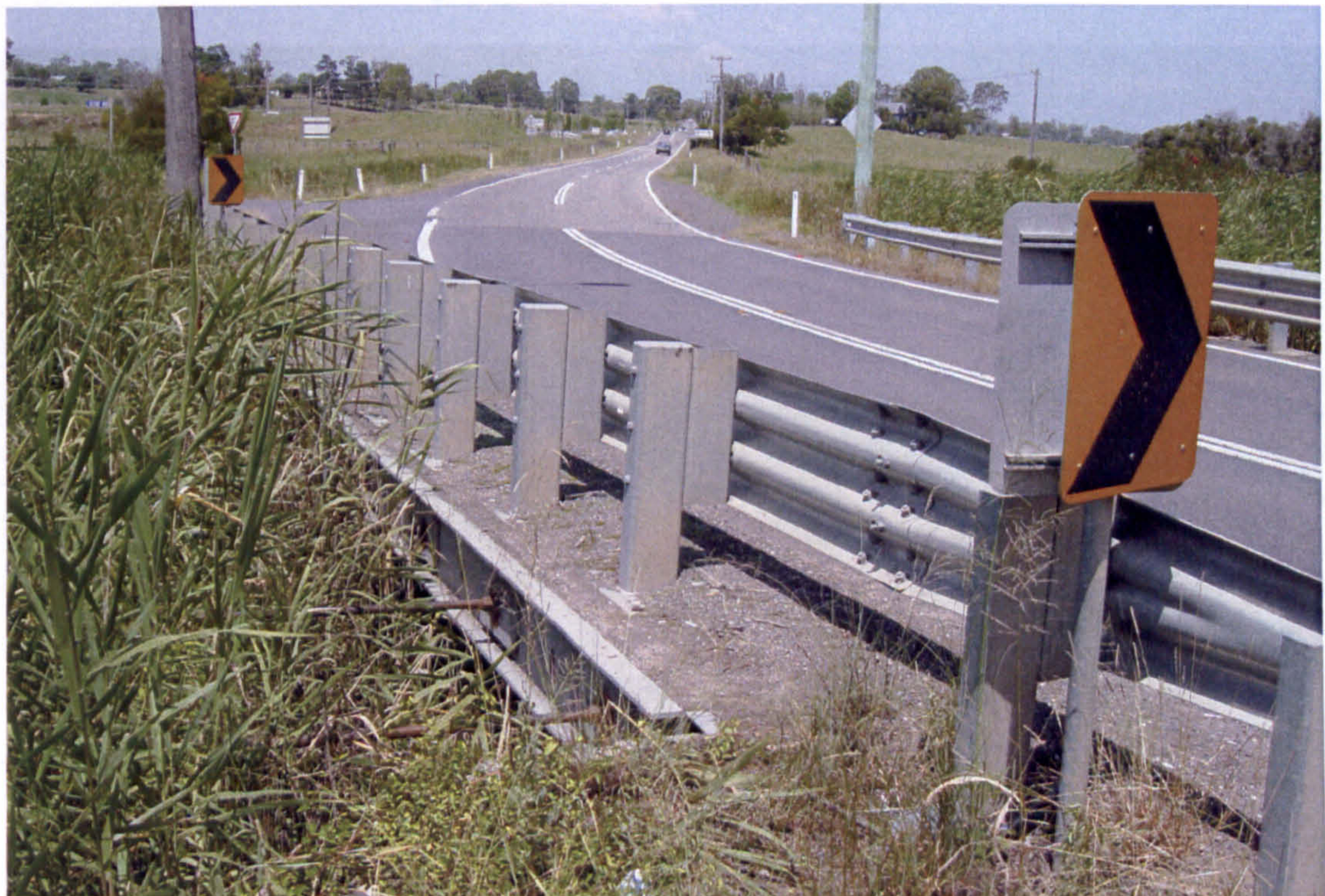
AUS - Extended bars for restressing – Continuous channel to spread concentrated load Sufficient resistance can be achieved to support a crash barrier
