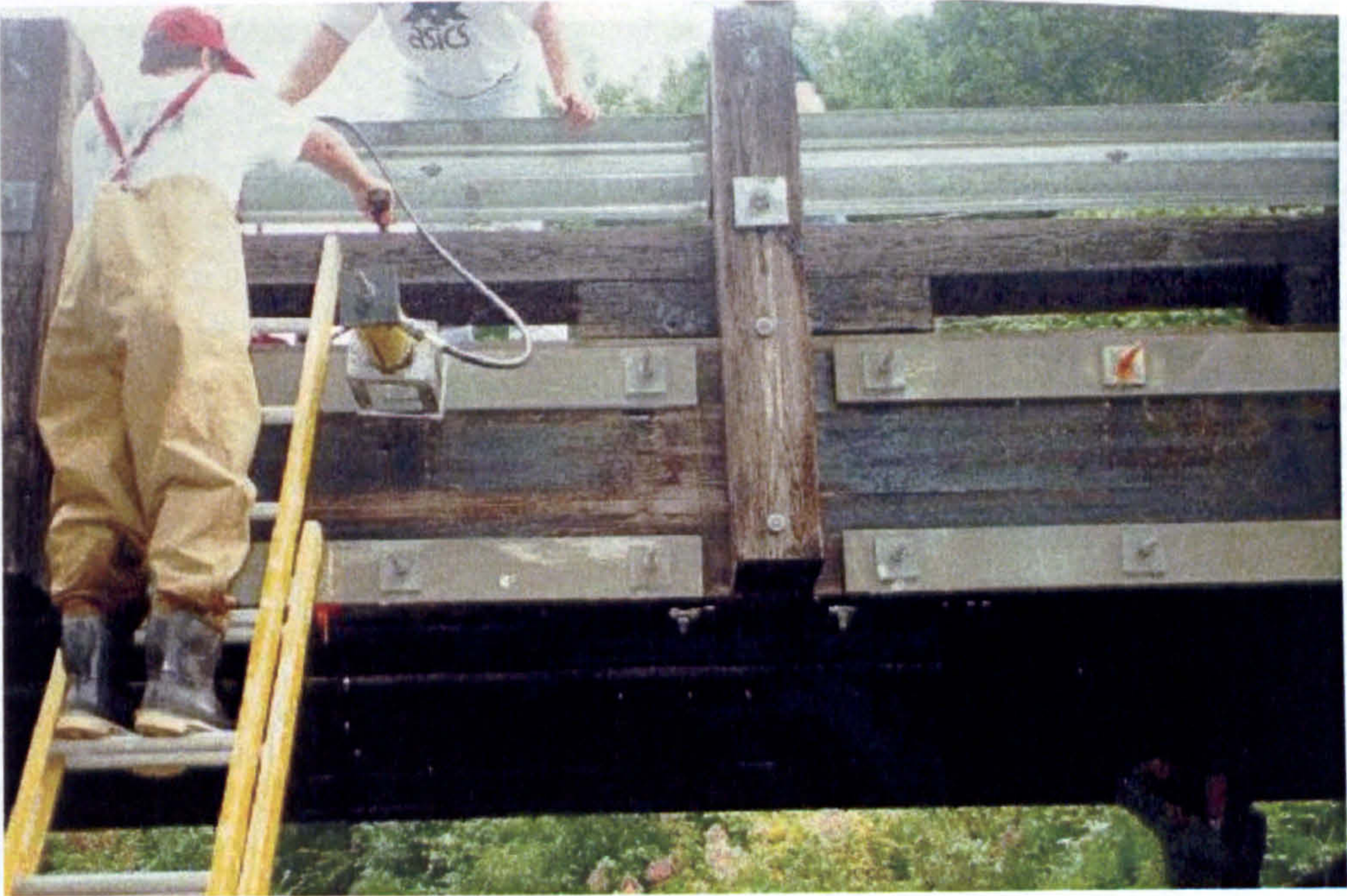
USA – Restressing of SLT deck
