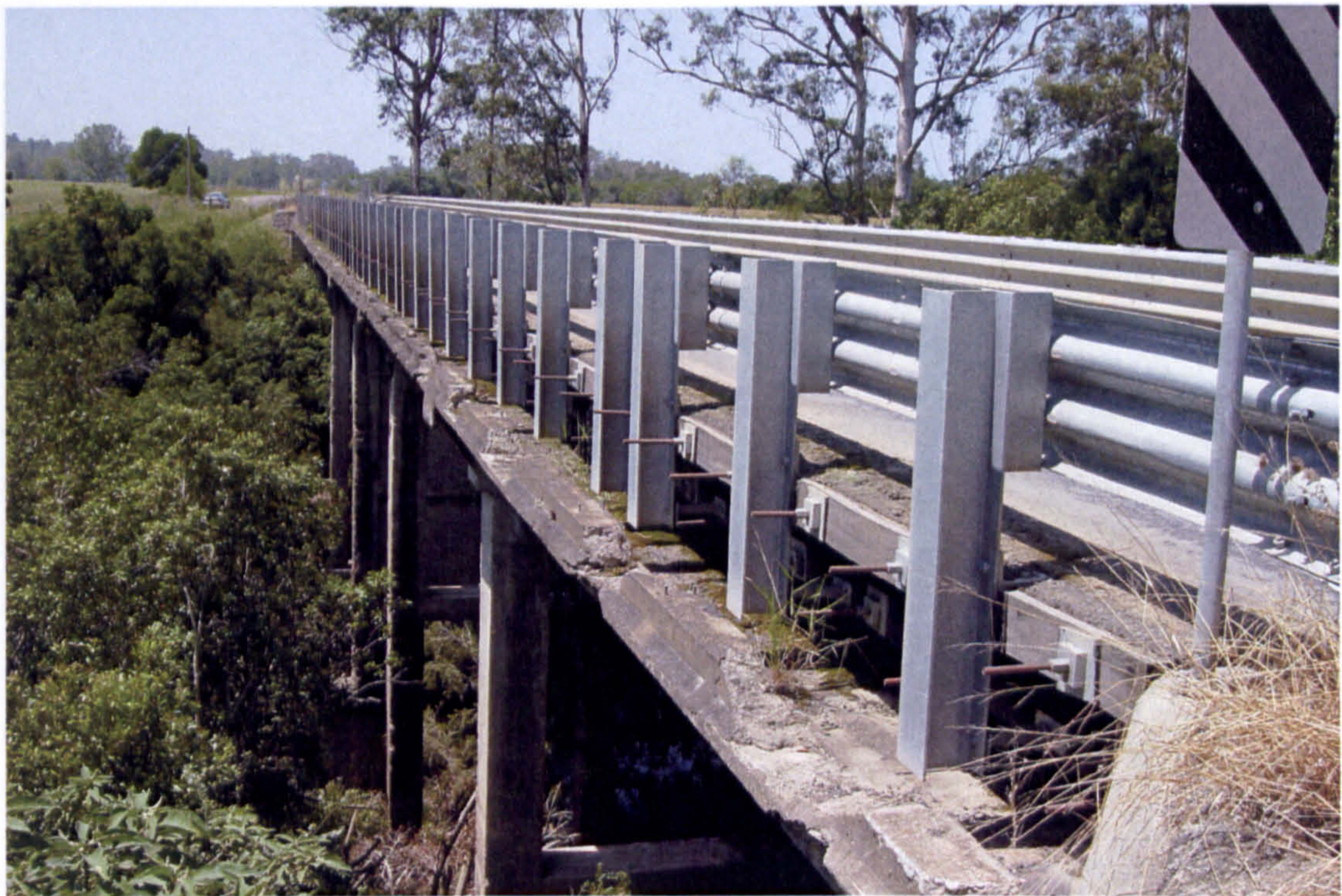
AUS - SLT deck laid over failed existing deck and using existing piers and abutments
