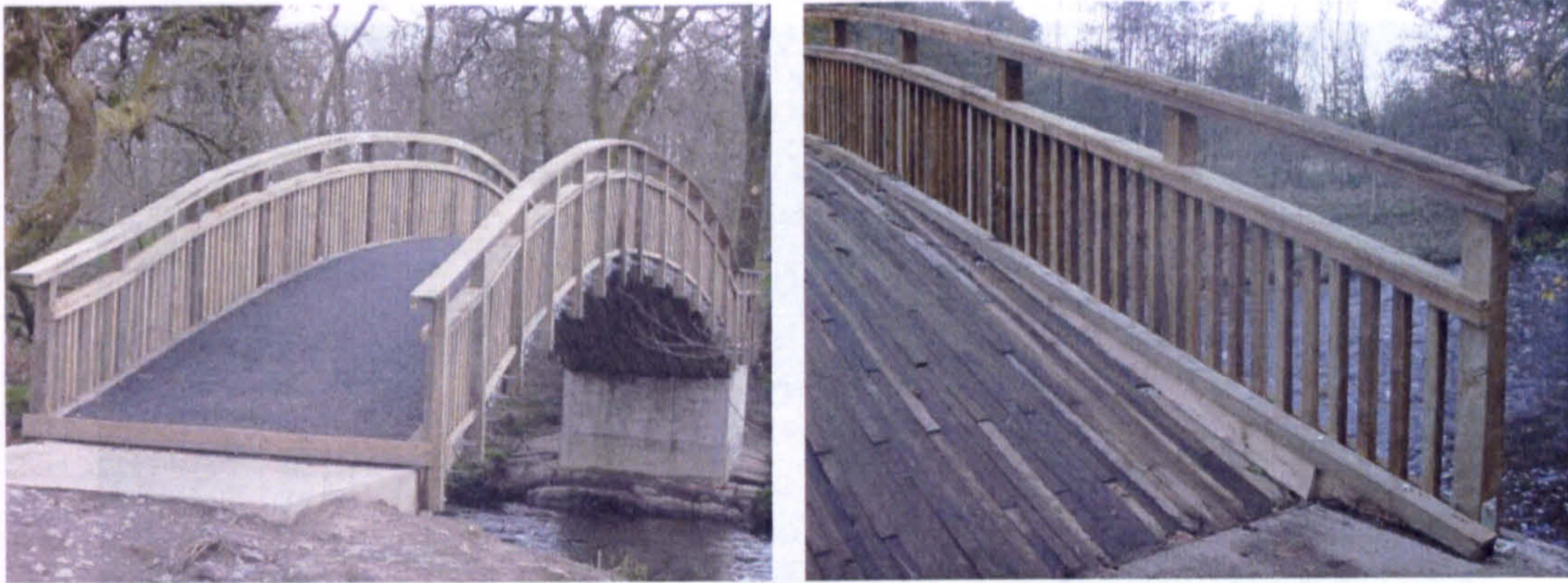
Fig 6.3 - Details of end of deck and tar
