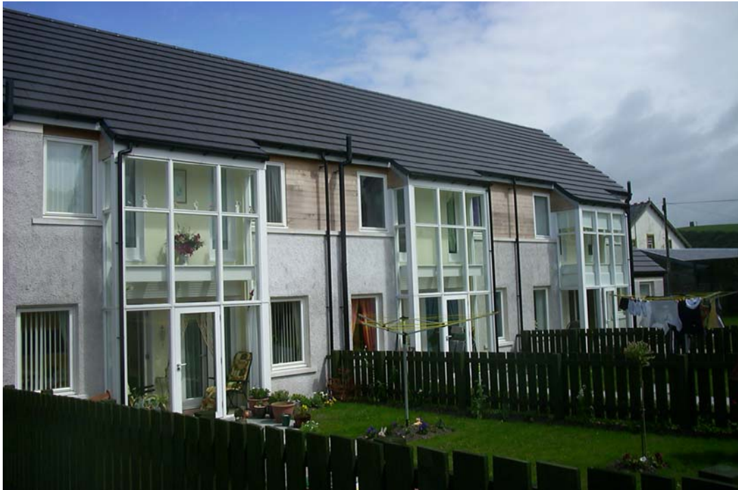
Fig. 1. Sunspaces installed on south façade of dwellings
