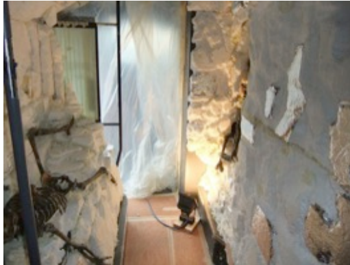
Figure 6.17. GGT crypt construction
