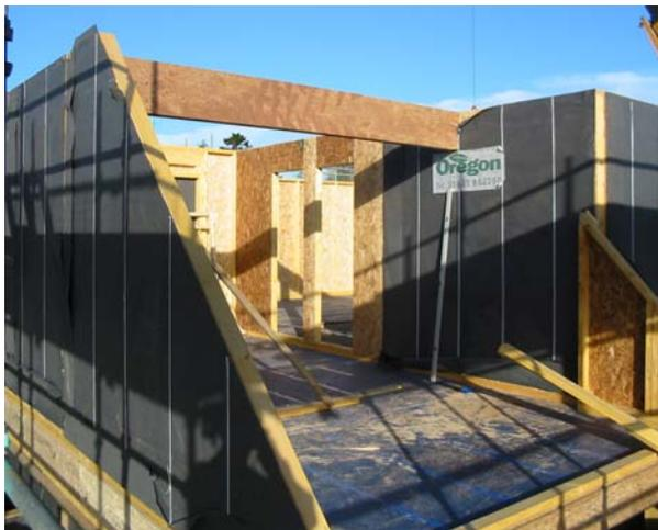
Figure 1: Timber platform frame during construction
