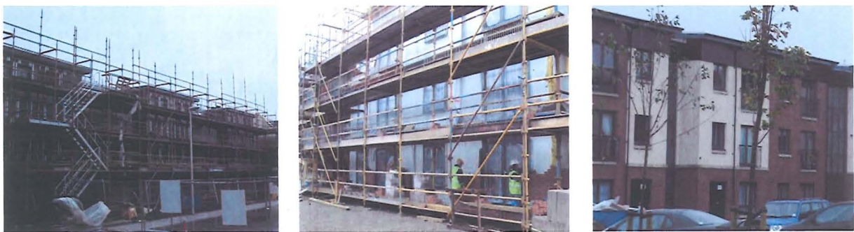
a) 3 Storey timber platform frame
