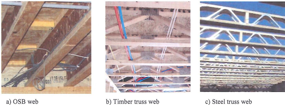
Figure 2.14 Examples of timber I-joist flooring systems
