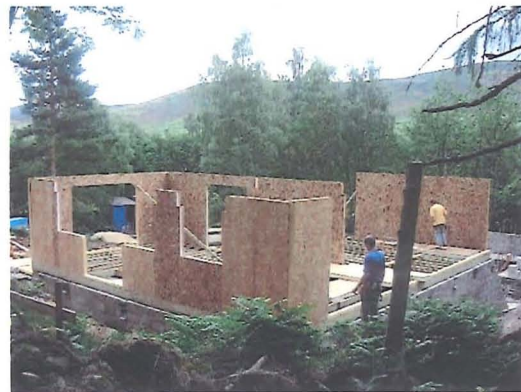
b) SIPs panels being erected
