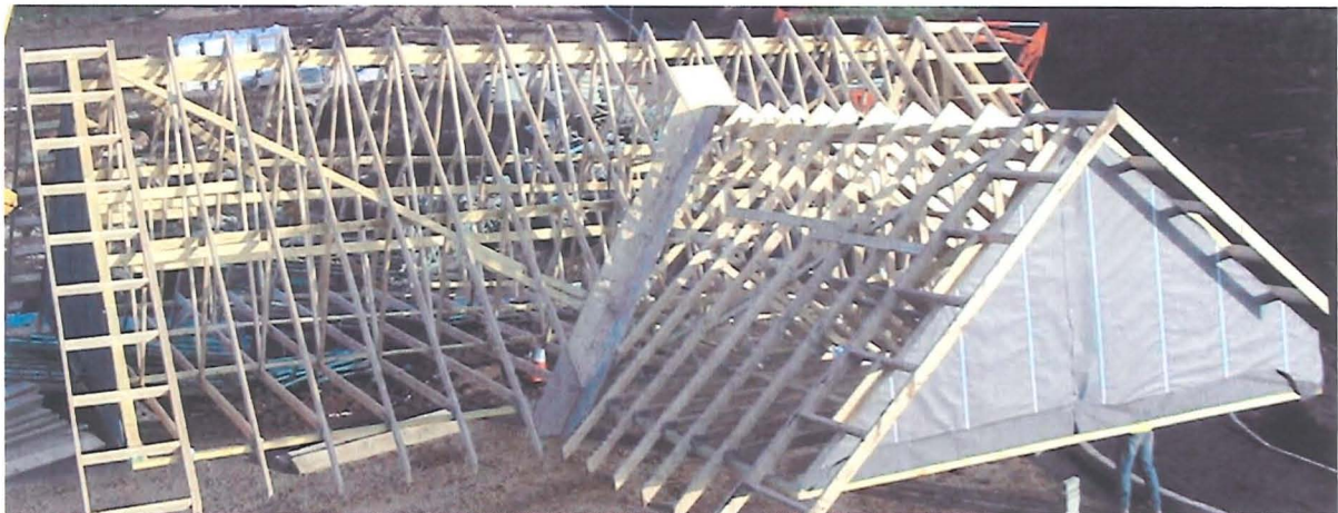
c) Truss rafter roof system
