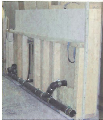
b) Insulated sanitary ware being fitted
