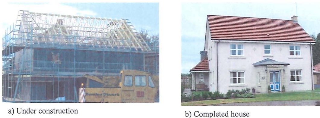
Figure 2.8 Standard two storey UK timber frame house
