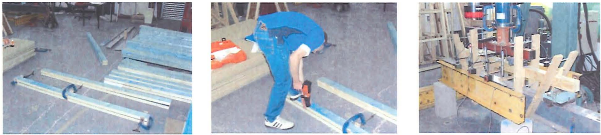
a) Fabrication and testing of fitch beams
