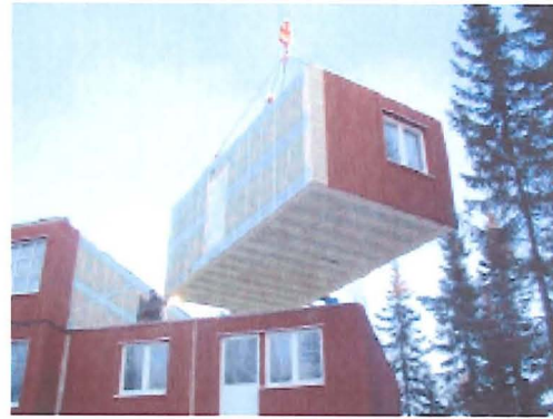
b) 3 dimensional timber modular unit (Stehn, 2005)
