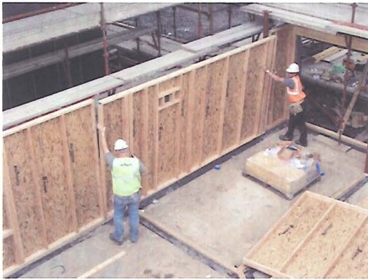
c) Ground floor panels erected
