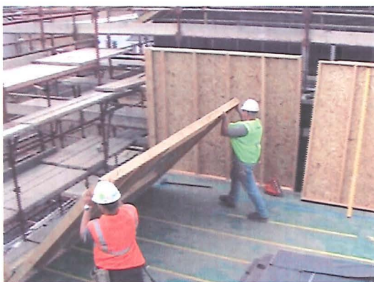
e) 1 st floor panels installed
