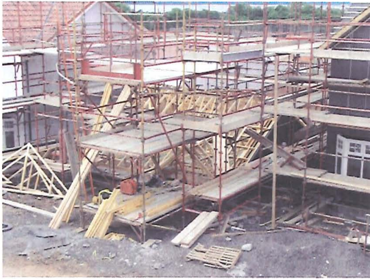
a) Roof constructed on ground floor slab
