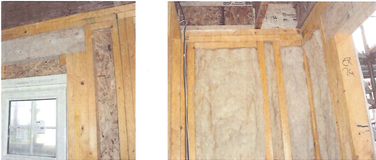
Figure 5.13 Examples of cripple studs supporting lintels
