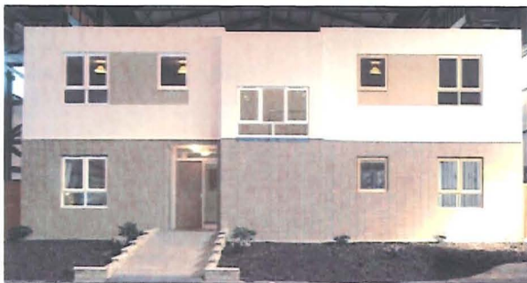
c) Demonstration building using mixed steel panel and modular construction (Lawson et al, 2005)
