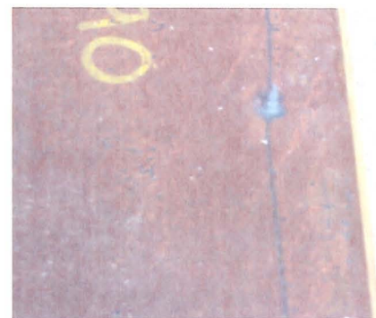
c) Pointside of nail after removal of timber showing cold weld
