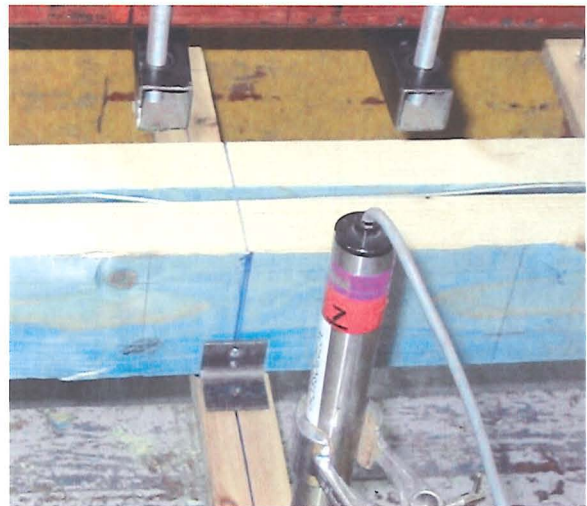
d) Buckling of steel in the top chord of an C24 strength timber fitch beam
