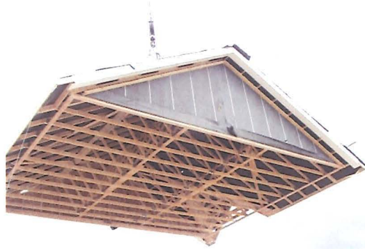
b) Roof lifted out of position
