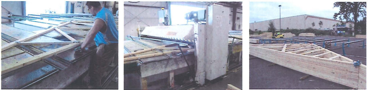
a) Placing of connection plate
