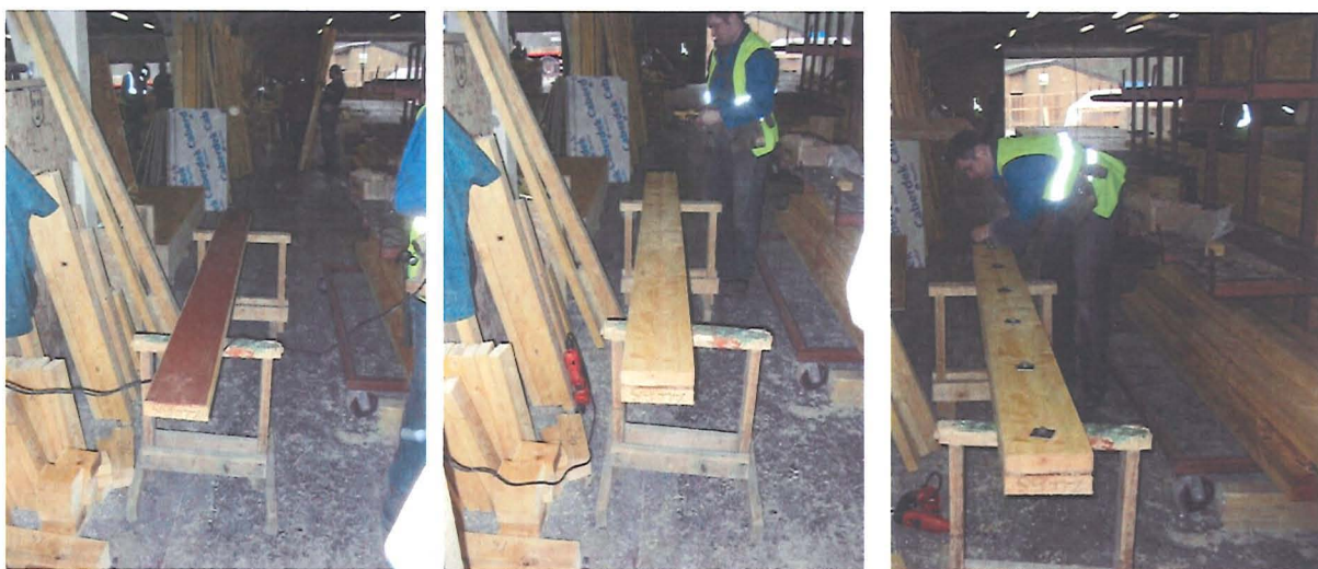
Figure 6.2 Fabrication of a bolted flitch beam
