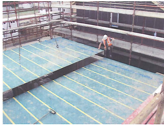
d) Cassette flooring installed
