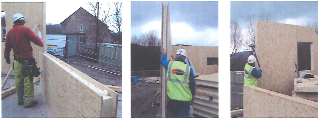
Figure 5.14 Structural Insulated Panels (SIPs) during construction
