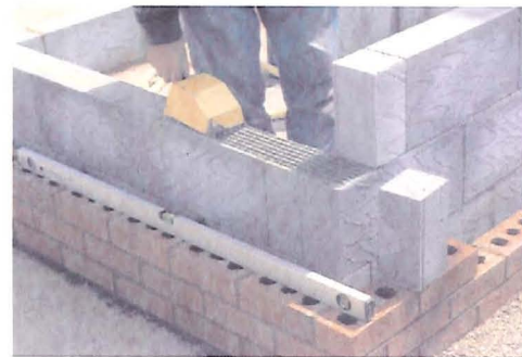
d) Thin joint block work (Thermalite, 2005)
