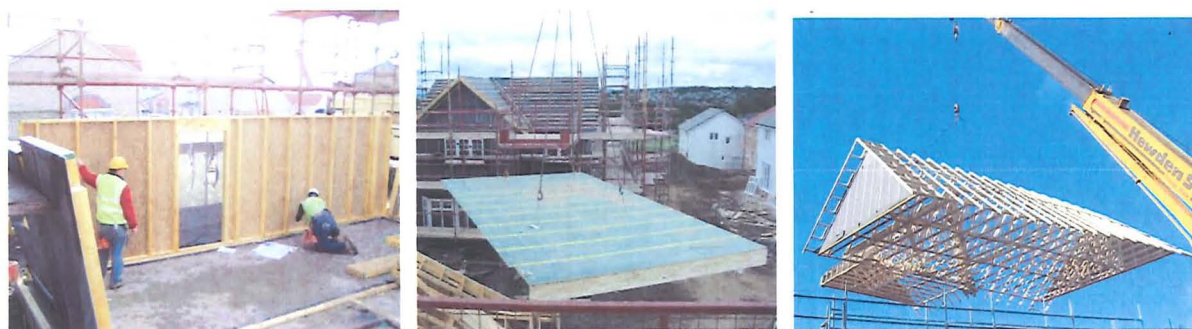
a) Wall panels
