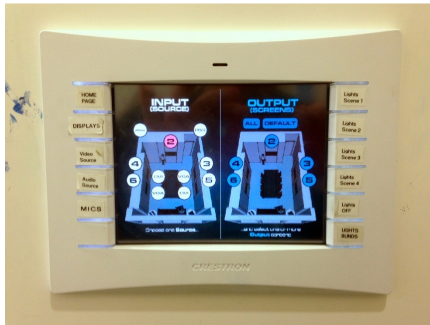
Figure 4 the Crestron™ interface for the configuration of the ICE. On the left, the zones as input sources, on the right the output screens.
