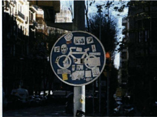
Figure 3.13: Stickers which damaged the pictogram of a sign.
