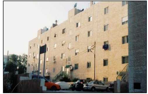
D. The North West Elevation
