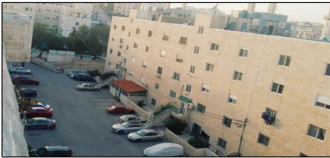
C. The Top View of the Compound Building Roof
