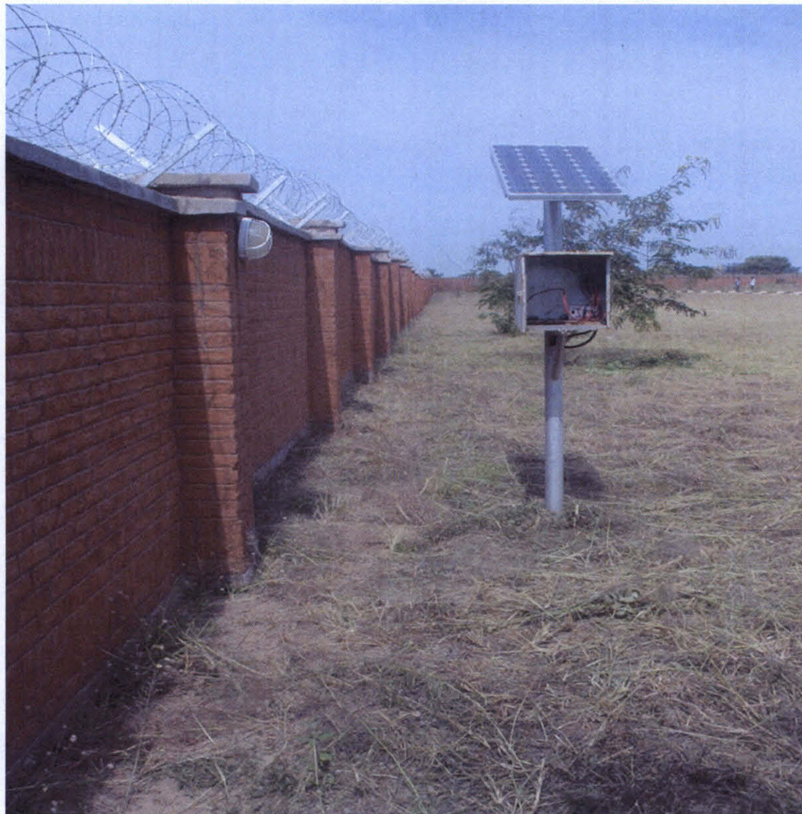
Figure 17: Solar panel at a remote secondary school
