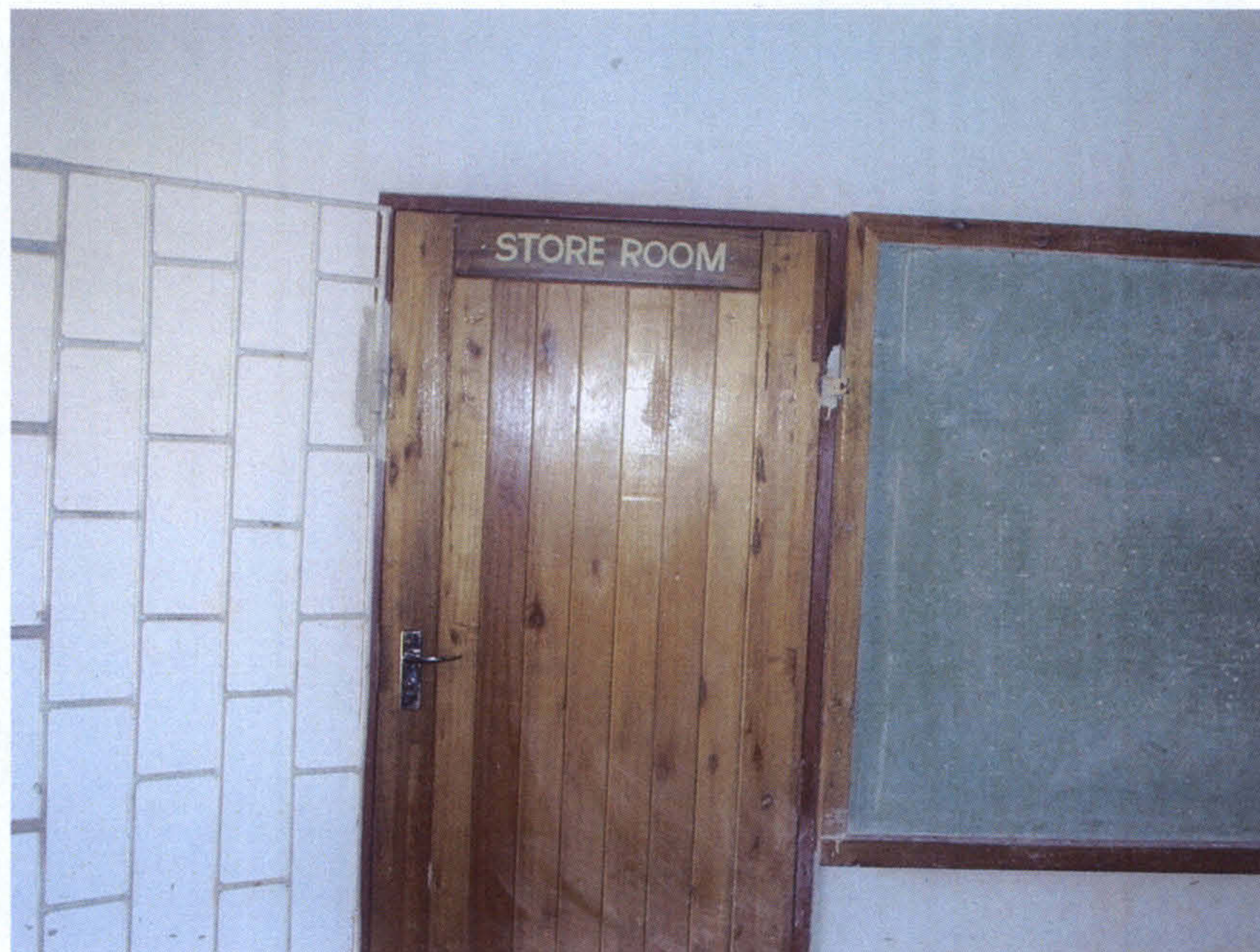
Figure 11: Storeroom with newly fitted burglar bars to protect computers
