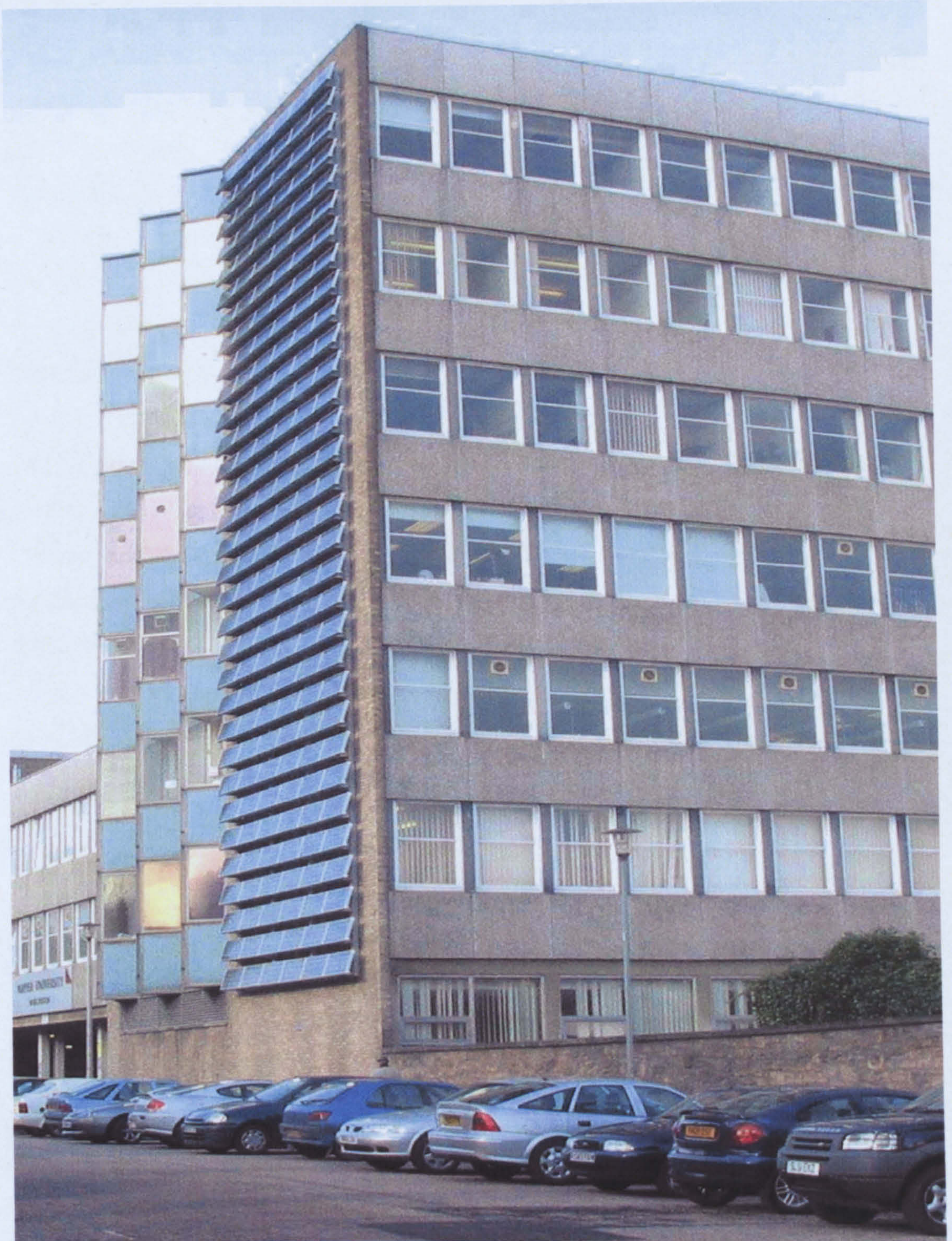
Figure 2.3.1 Edinburgh Napier University solar facade under discussion.
