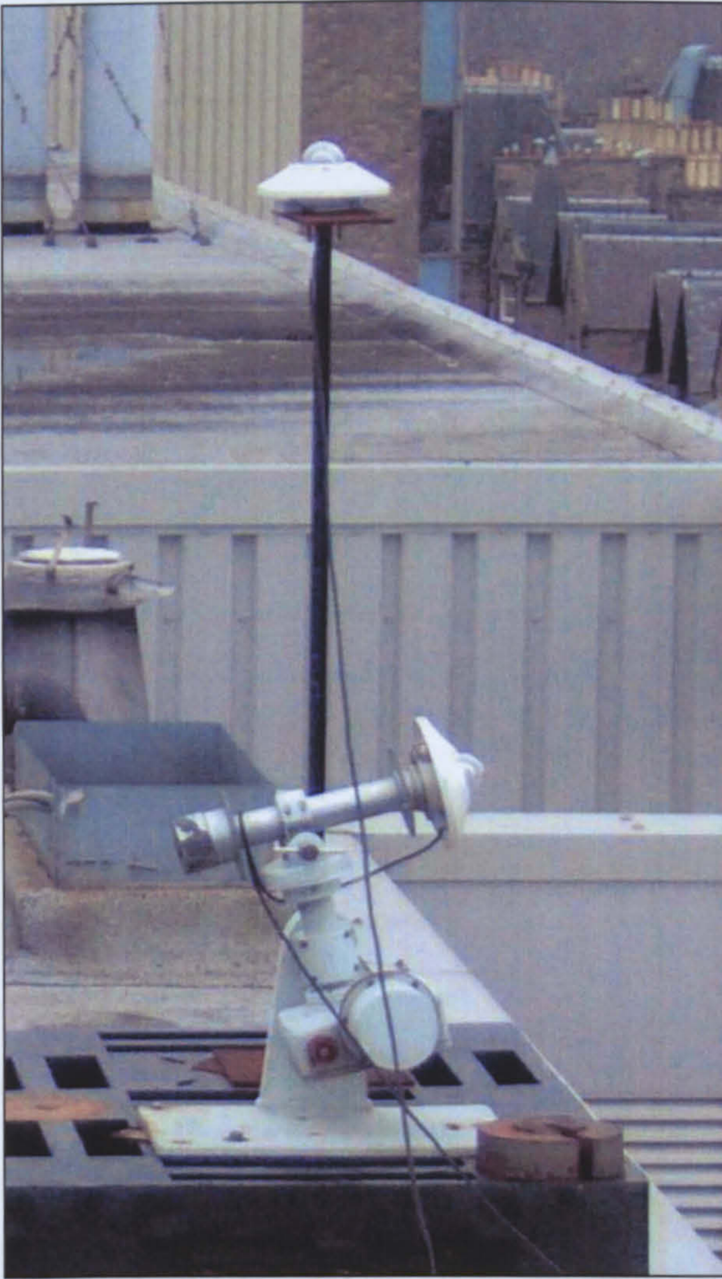
Figure 3.4.2 Horizontal and inclined pyranometers installed at new location on the rooftop of Edinburgh Napier University to record solar irradiance for the current study.
