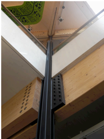
Figure 4: Column flitch plate connection (Image copyright: Buro Happold)
