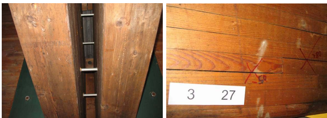
Figure 2: Main beam of roof structure (left) and crack in glue-line (right)
