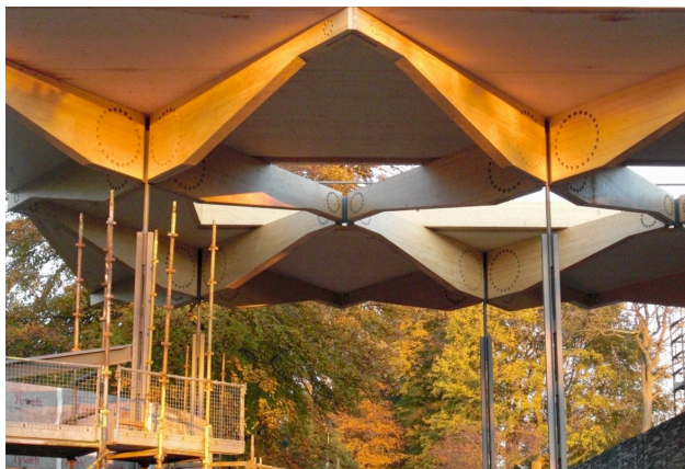
Figure 7: Roof construction over entrance lobby (Image copyright: Buro Happold)
