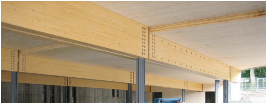
Figure 3: Cross-laminated panels spanning between glulam beams (Image copyright: Buro Happold)
