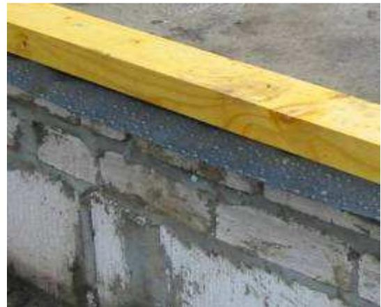
b) Typical sole plate to 7N/mm<sup>2</sup> concrete brick wall footing connection
