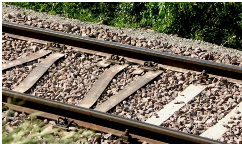
Figure 8-13 Y-sleepers allowing a reduction of the clearance profile
