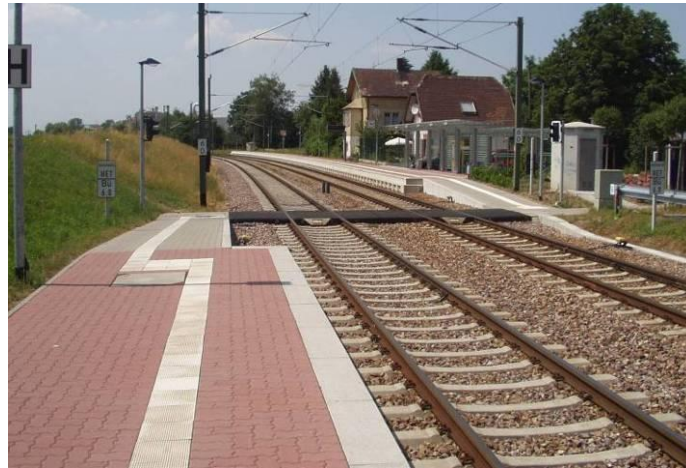
Figure 8-18 Standard layout of platforms for TramTrains
