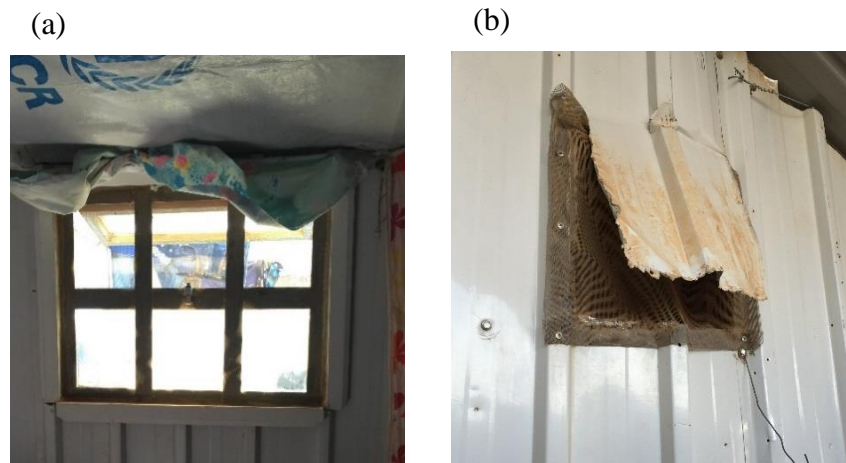
Figure 5.10: Azraq camp ventilation openings: a) The small window in the T-shelter, b) An opening opened in the wall by the residents
