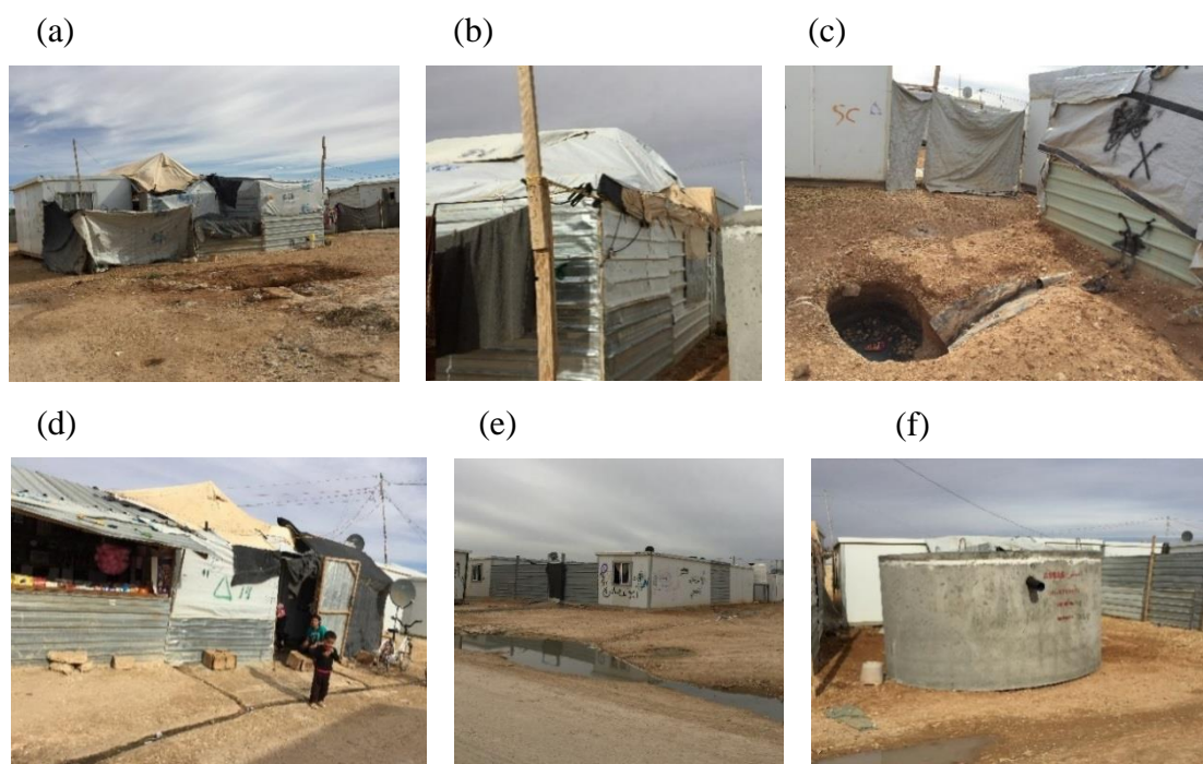
Figure 4.18: Facilities: a) Outdoor facility with a nearby pit, b) Canvas roof over a toilet, c) Wastewater ditch and pit, d) Network of surface runoff wastewater, e) Surface runoff wastewater, f) Concrete tank to be installed
