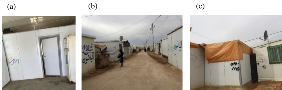
Figure 4.7: Zaatari camp floor adjustments: a) A concrete floor replacing the wooden floor, b) A street view showing how the residents filled the underneath of the shelters with earth, c) A shelter's raised floor being filled with earth
