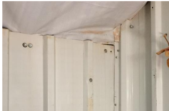
Figure 5.8: A junction between two steel sheets in the wall and the plastic sheeting roof
