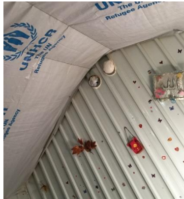
Figure 5.7: Blocked ventilation pipes to limit the dust ingress
