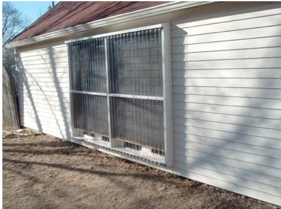
**Figure 1.6: Solar air systems for preheating air in a garage.**
