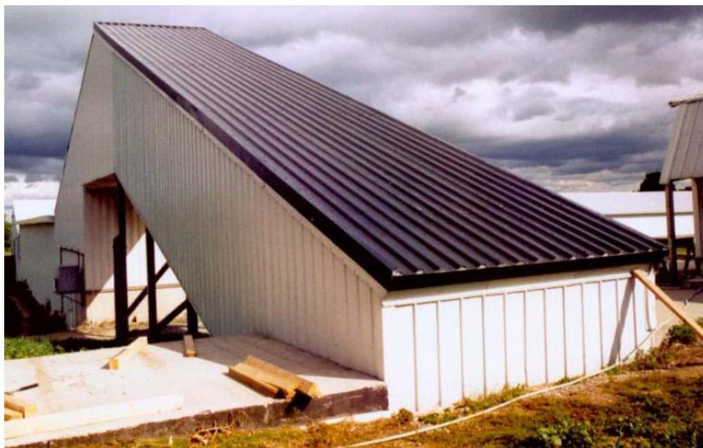
**Figure 1.7: Roof mounted Solarwall installation.**
