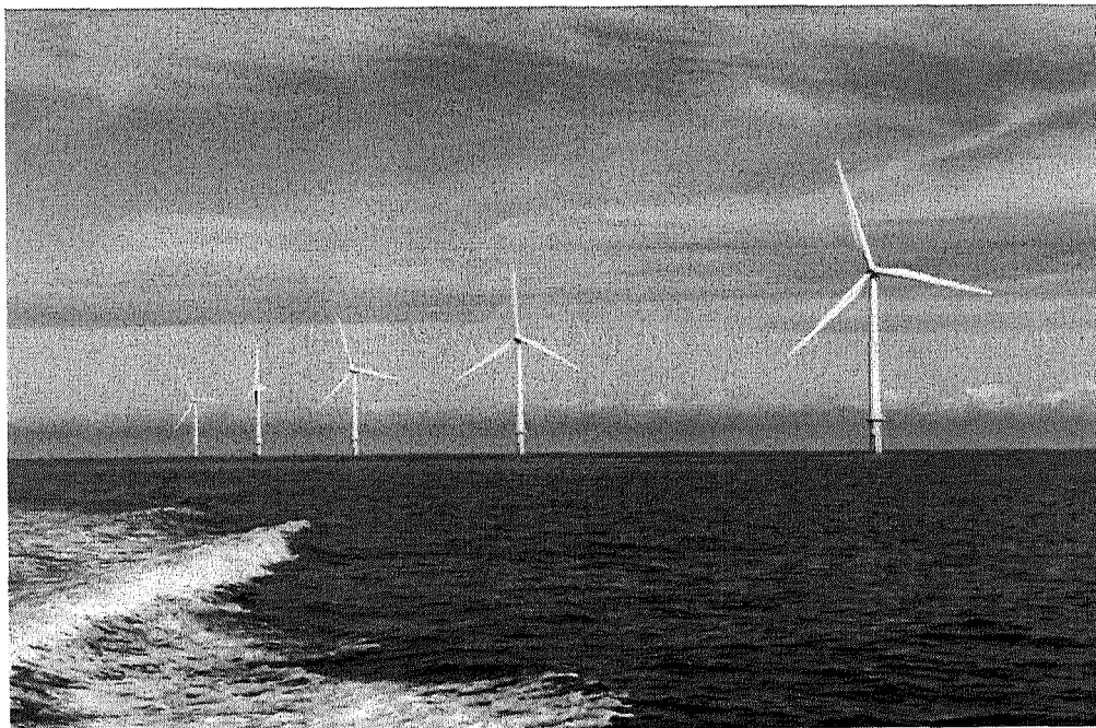
Figure 5.8 Wind turbines at the operational Burbo Bank offshore wind farm (Trine Hoffman Sørensen 2010)
