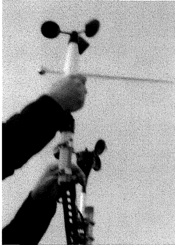
Figure 3.8 Installation of Vaisala WM302 and NRG #40H anemometers on the roof of Merchiston campus
