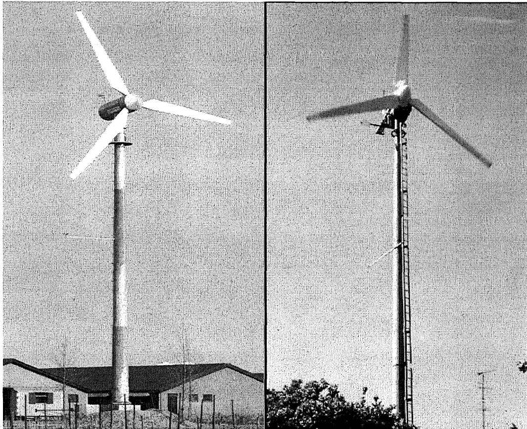
Figure 5.1 On the left 15KW downwind turbine and on right 22KW upwind turbine (Winds of change 2010)
