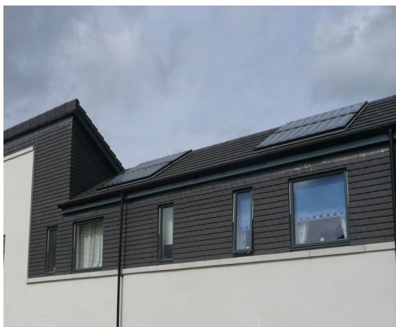
Plate 6 Solar Hot Water Installation
