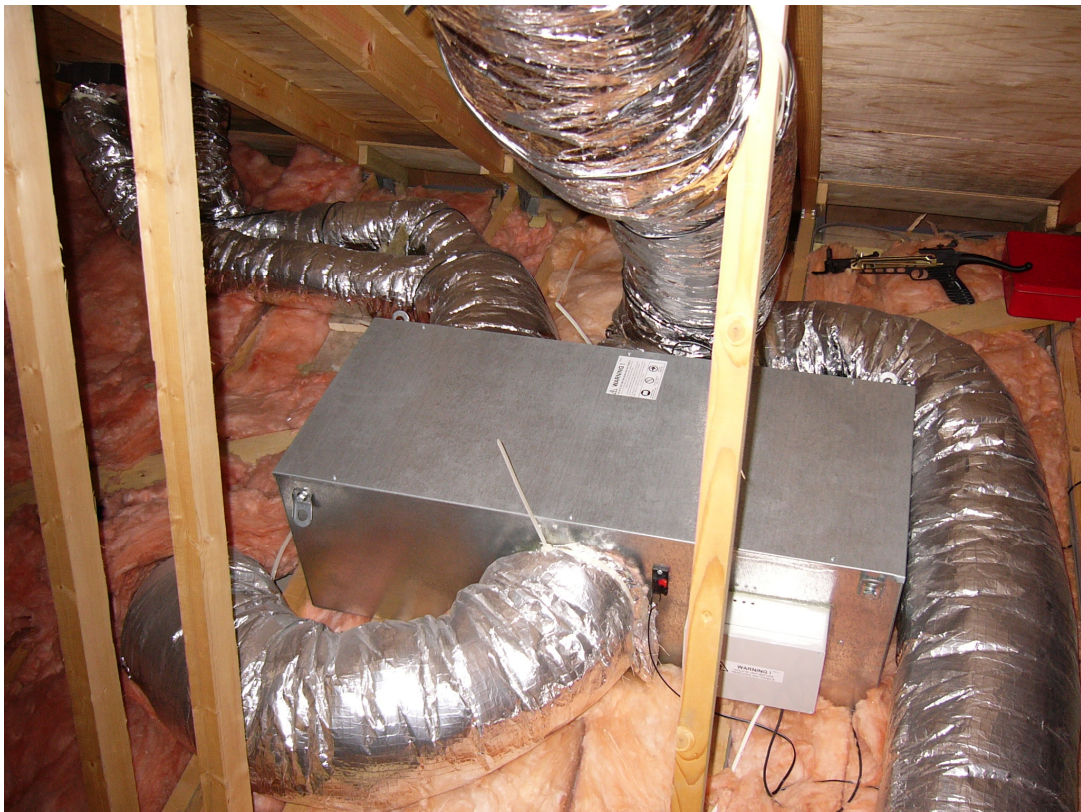
Plate 8 NuAire Positive Input Ventilation System
