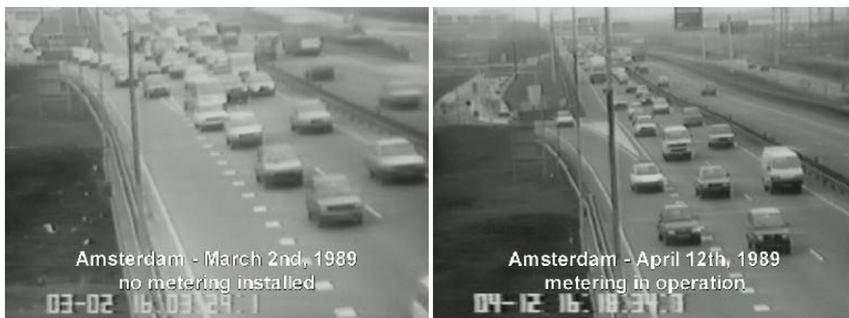
Pre-ramp metering mainstream merging (left) and with metering in operation (right) in the same Amsterdam ring-road on-ramp.
