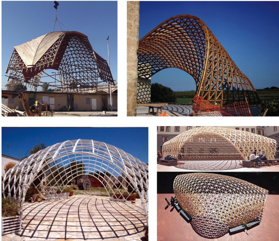
**Figure 18:** Post-formed timber grid shells [16].
