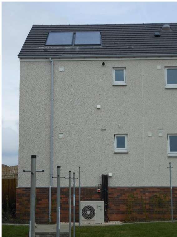
Figure 3: (left) Diversity of heating technology - ASHP & Solar Thermal
