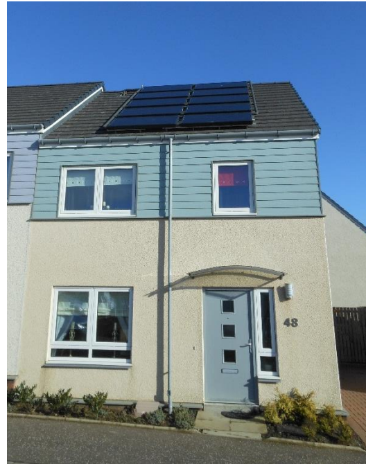
Figure 7: Block 9 - CCG terraced dwellings
