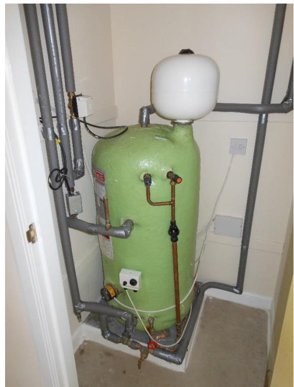
Figure 4: (right) Water cylinder for ASHP
