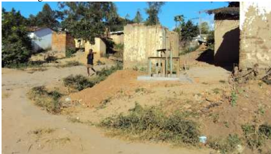
Figure 2. New kiosk under construction in Golio THA
