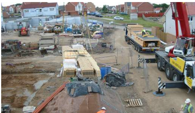
A) LOOSE MATERIAL SENT TO SITE FOR FIRST FLOOR CONSTRUCTION
