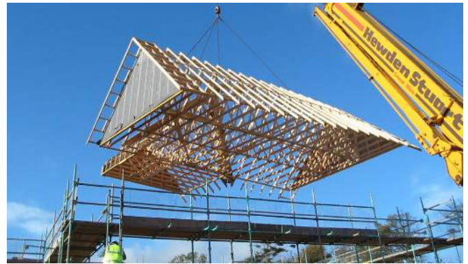
FIGURE 16 STRUCTURAL PERFORMANCE – APPLIED ACTIONS DURING LIFTING
