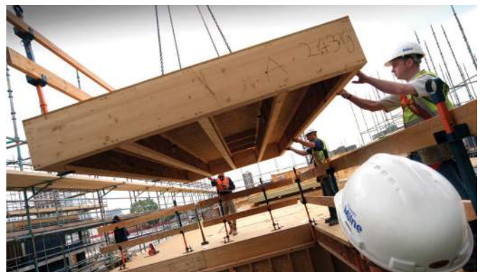
B) LANDING OF A PREFABRICATED FLOOR CASSETTE
